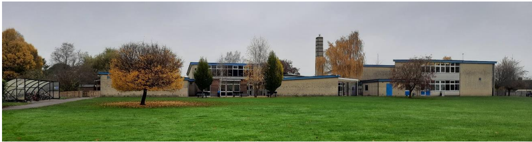
VIEW OF EXISTING SCHOOL BUILDING FROM SOUTHERN PLAYING FIELD
