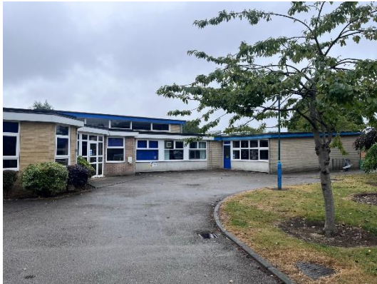
VIEW OF SCHOOL ENTRANCE
