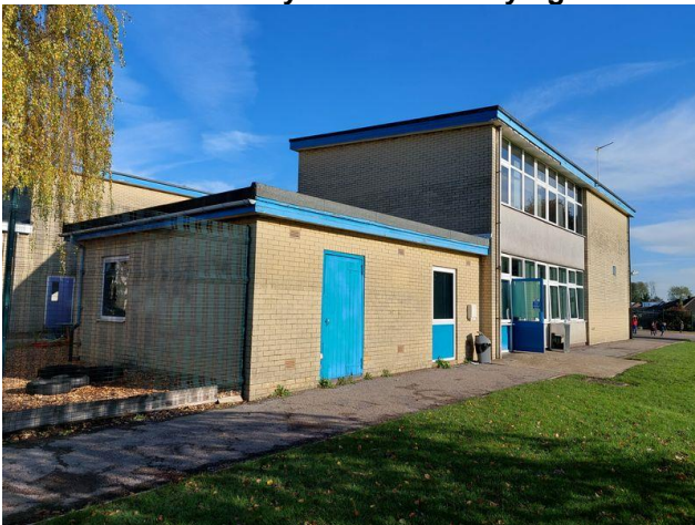
Plate 9.3: Main School Building
