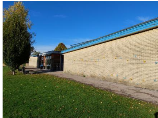
Plate 4.6: Western end of southern elevation
