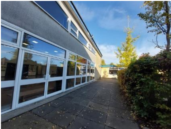
Plate 4.3: Central section of eastern elevation
