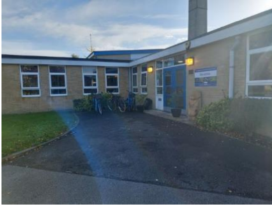
Plate 4.1: Main entrance, central section of northern elevation
