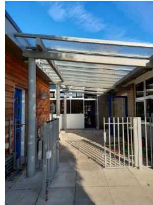
Plate 4.23: Canopy connecting the eastern elevation to the Main School Building
