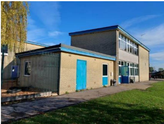
Plate 4.5: Eastern end of southern elevation
