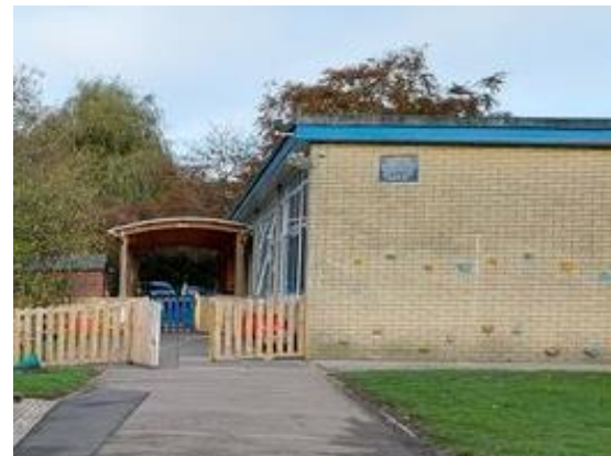
Plate 4.10: Canopy at northern end of western elevation
