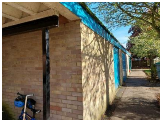
Plate 4.25: Storage room in centre of building
