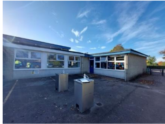
Plate 4.8: Western end of northern elevation
