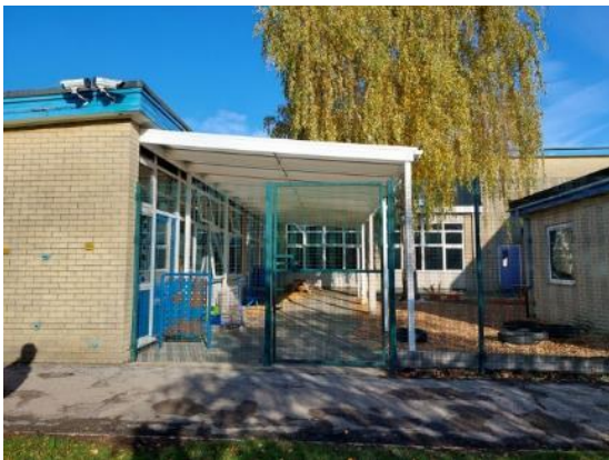
Plate 4.9: Courtyard in central section of southern elevation
