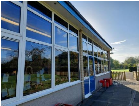
Plate 4.7: Southern end of western elevation
