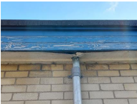
Plate 4.17: Damaged soffit
