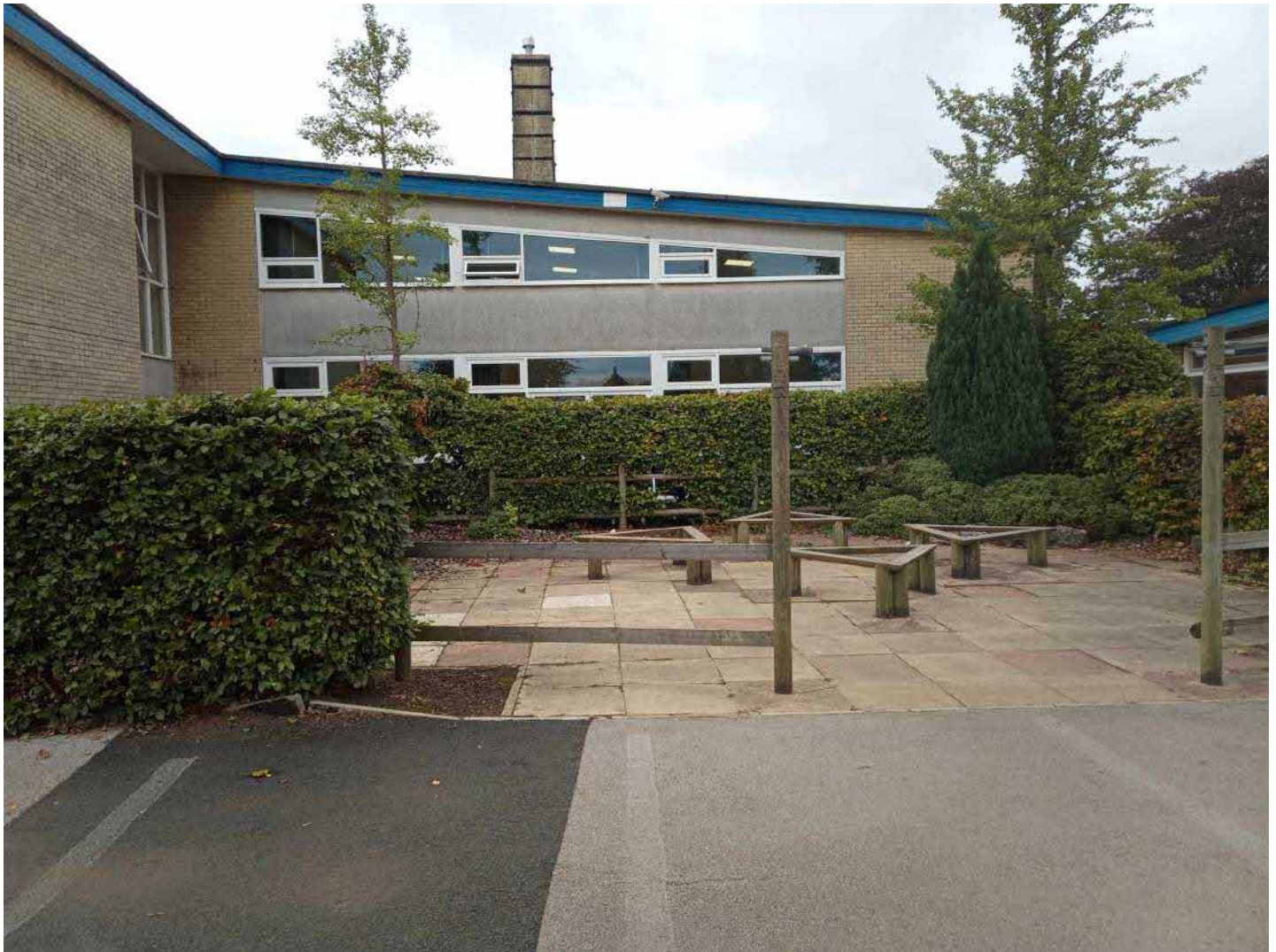
Location 09 facing West - Two storey section of EFAA building, Chimney and outdoor seating
