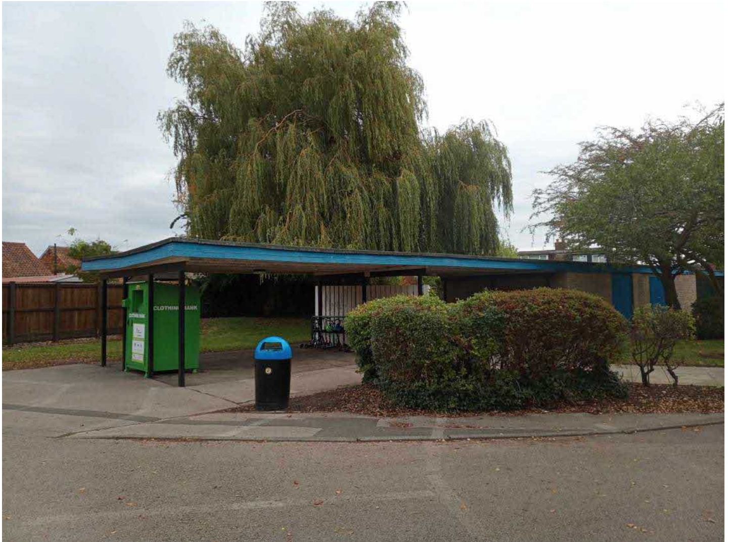
Location 02 facing North East - ANC1 Building
