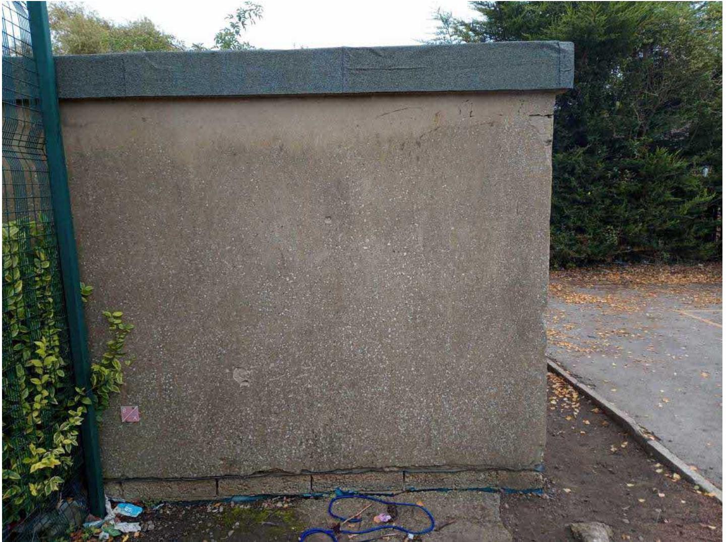
Location 11 facing South East - Shed
