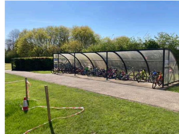
Cycle shelter to western side
