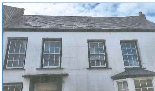
Eastern aspect as seen from Bank Street showing the other small roof
