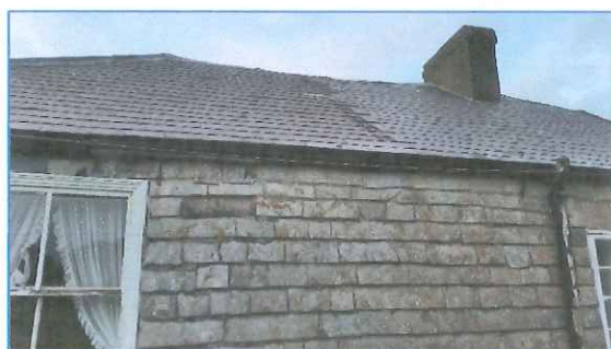
Larger hipped roof on the southern side of the building
