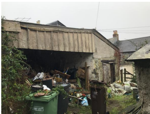
Front elevation with asbestos cladding
