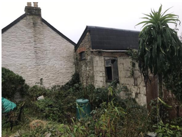
Rear west elevation with window
