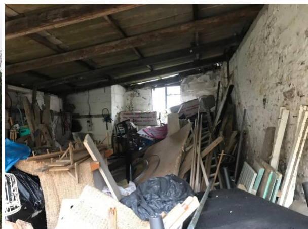
Roof structure and internal walls
