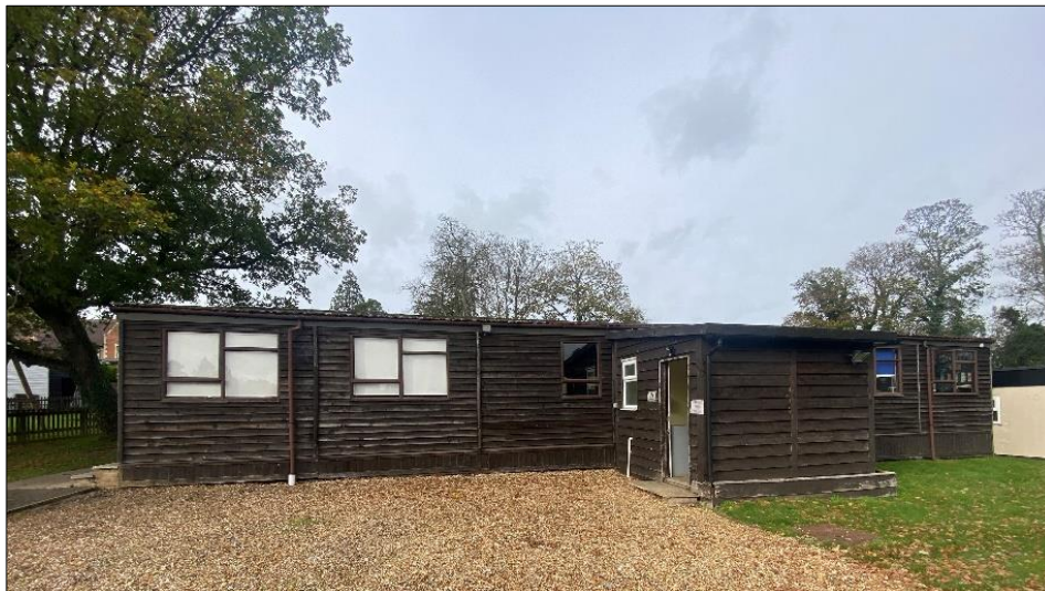
Existing east elevation of the temporary building
