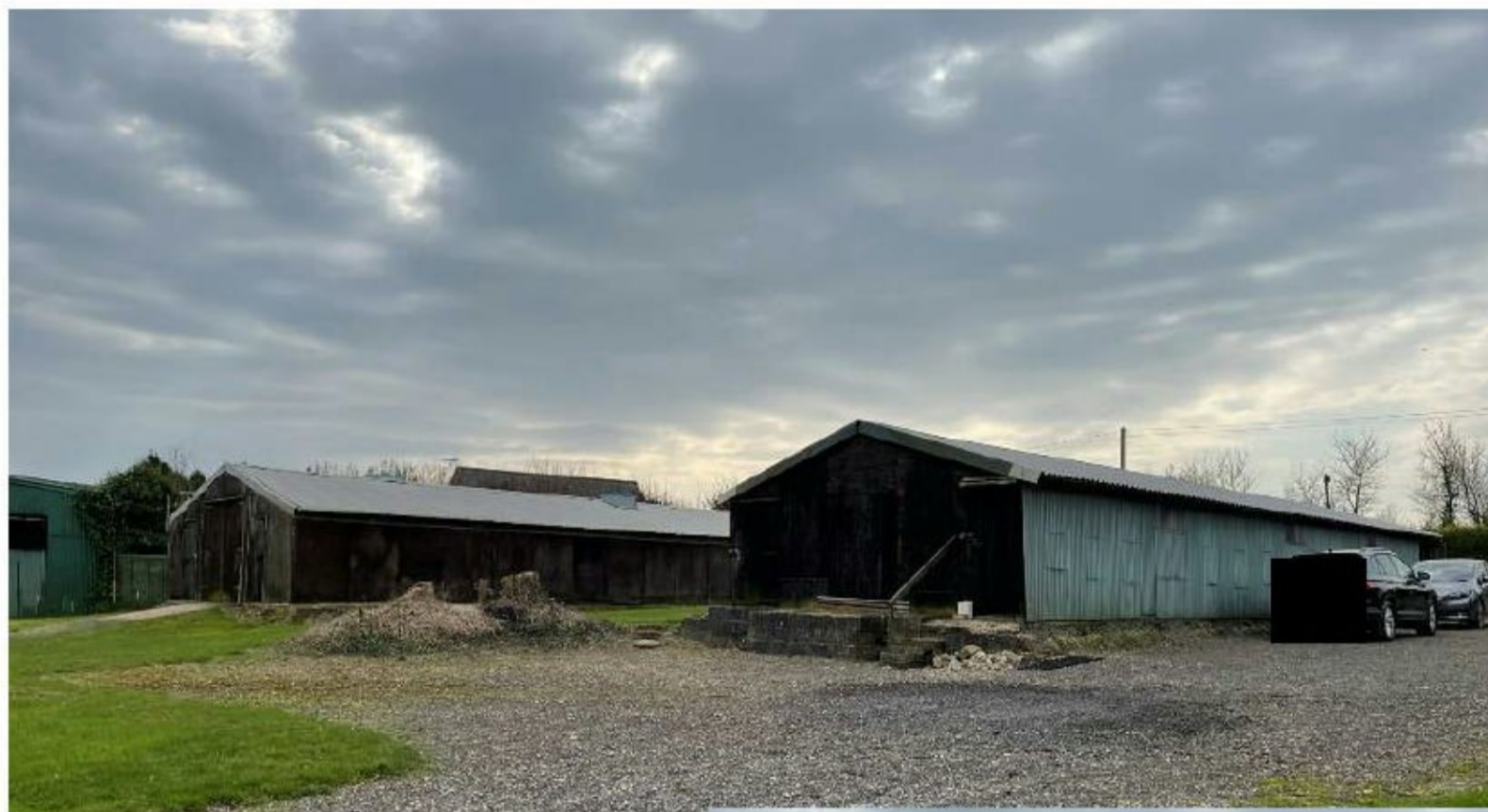
Left Photo - Building 2 (right) and building 3 (left) Photo Below – Building 3
