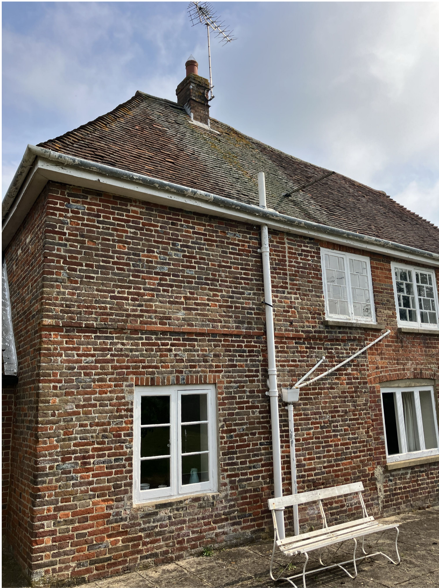
Image 1 Rear of house indicating existing SVP and waste pipes
