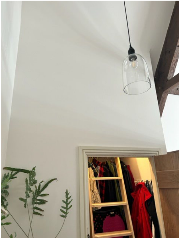
Photo 7: Entrance the larger roof cavity space above cupboard.
