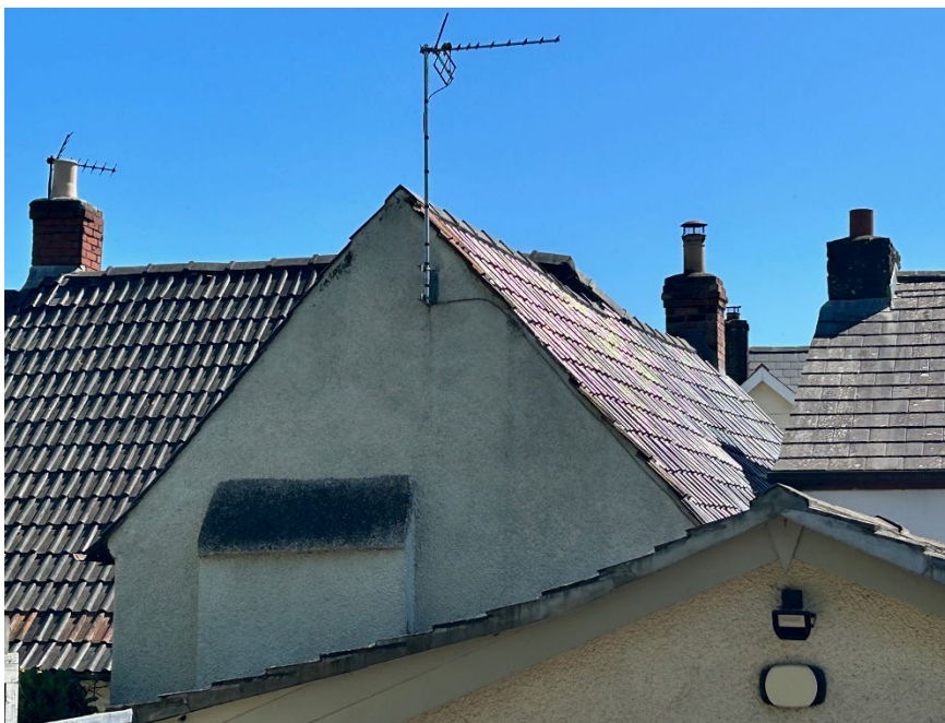
Photo 4: View of the back of the house / roof from the garden.
