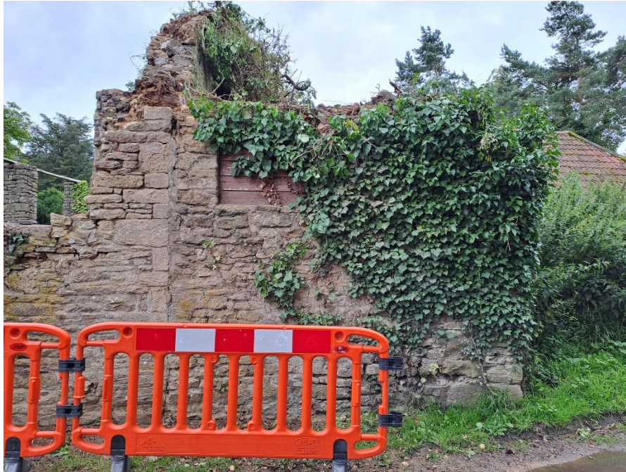
North wall after dismantling
