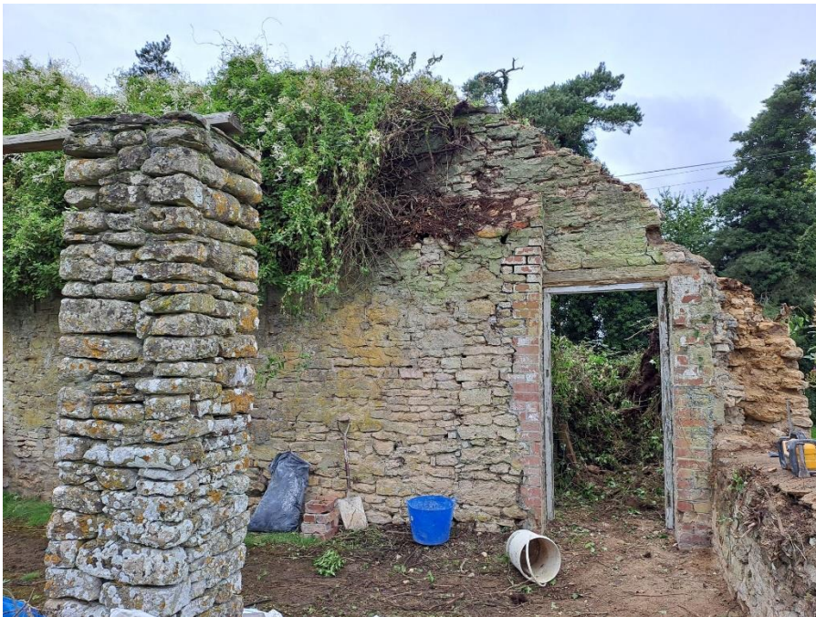
East wall after vegetation clearance and dismantling
