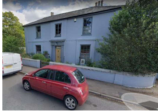
Front elevation of main property
