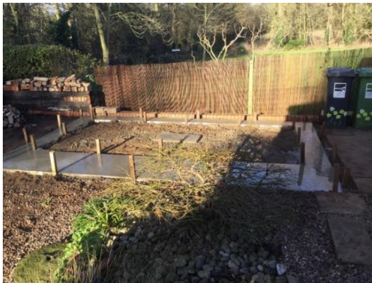
Example of a Ring beam (not to scale)
