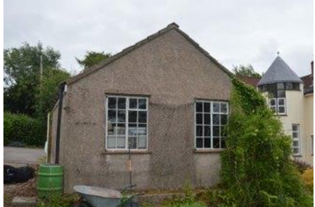
Photograph 17: View of gable end on the western elevation of the garage.
