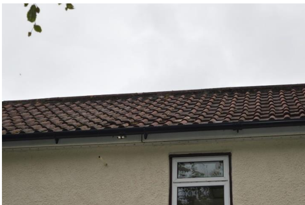
Photograph 11: Alternative view of the western elevation.
