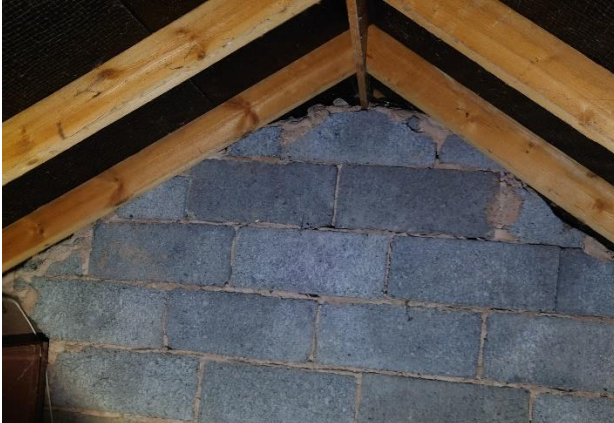
Photograph 16: Alternative view of roof void.
