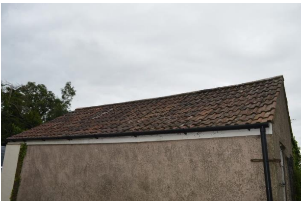
Photograph 18: View of north facing elevation on the garage.
