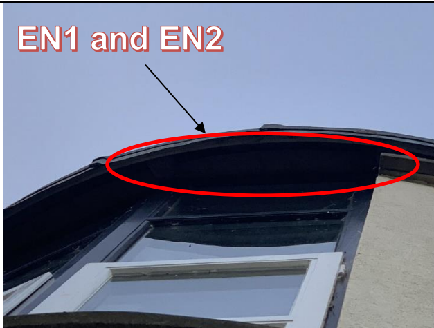
Photograph 7: View of the turret on the eastern elevation.
