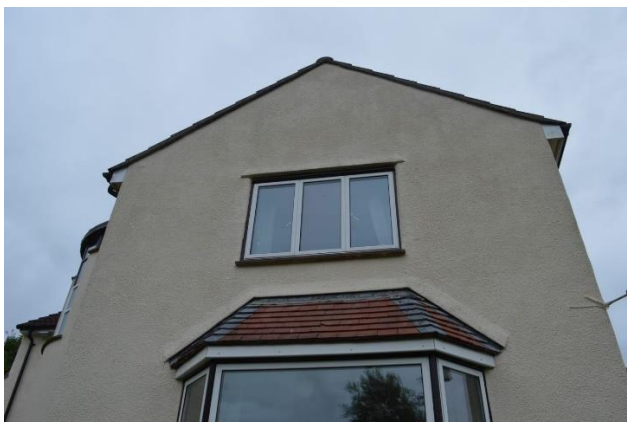
Photograph 9: View of the gable end on the eastern elevation.
