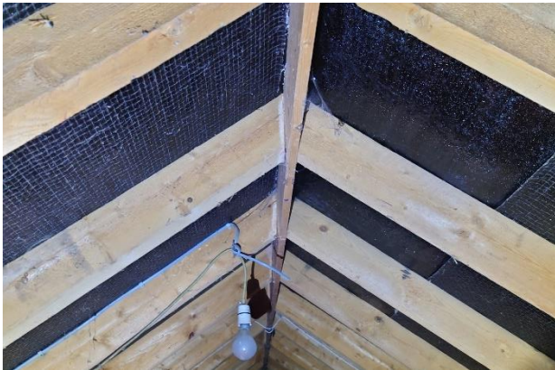
Photograph 14: View of roof void in house.
