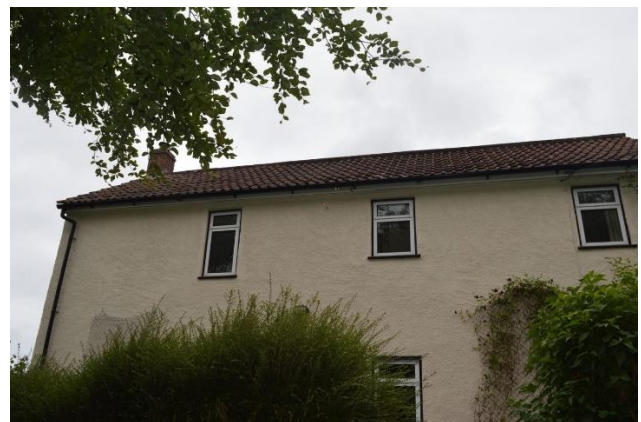
Photograph 10: View of the western elevation.
