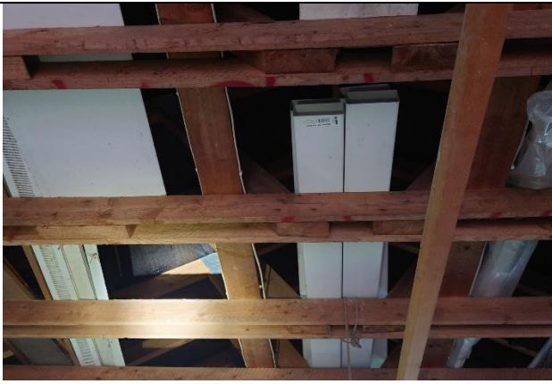
Photograph 20: Internal view of garage.
