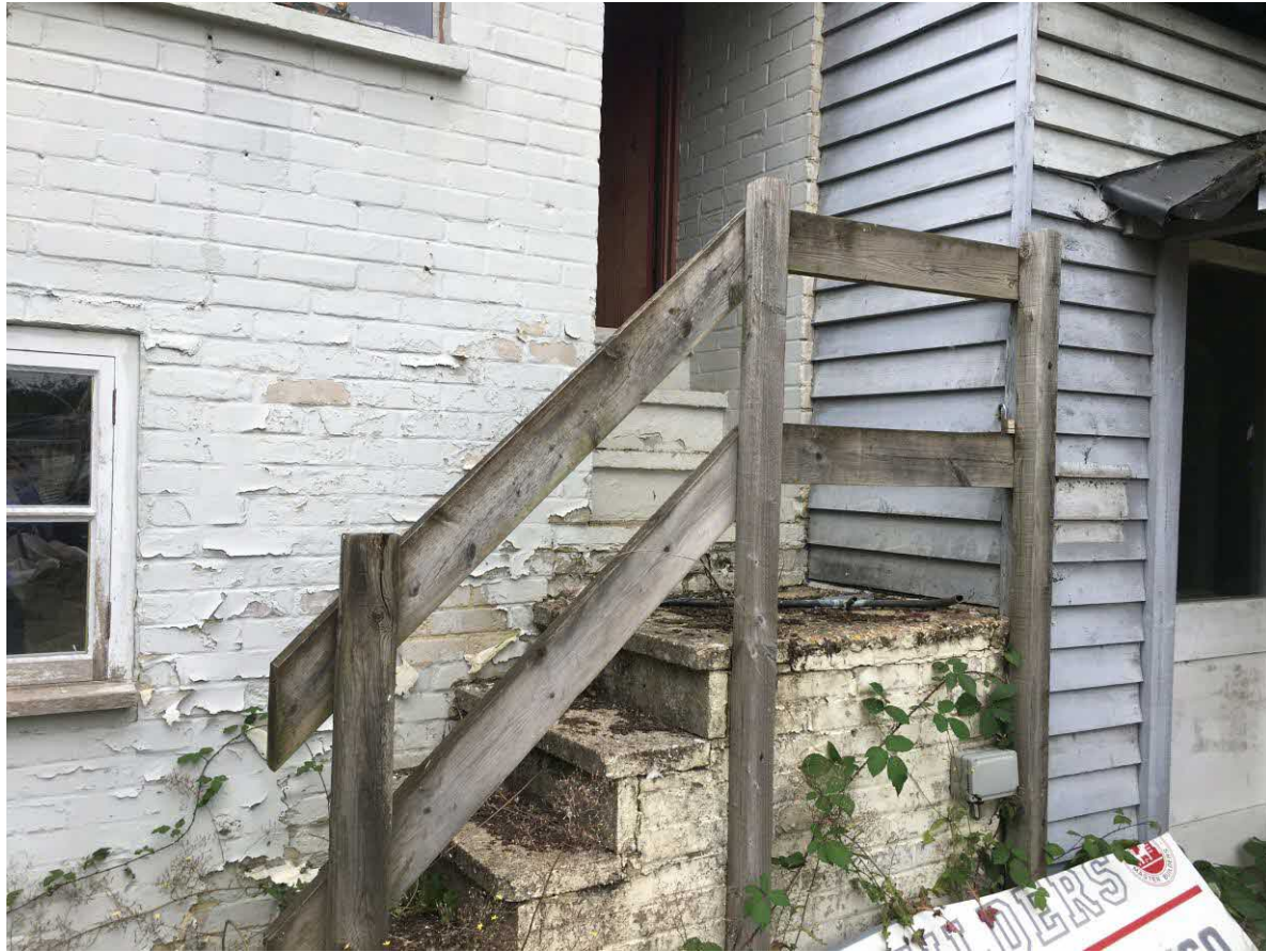
Access to first floor
