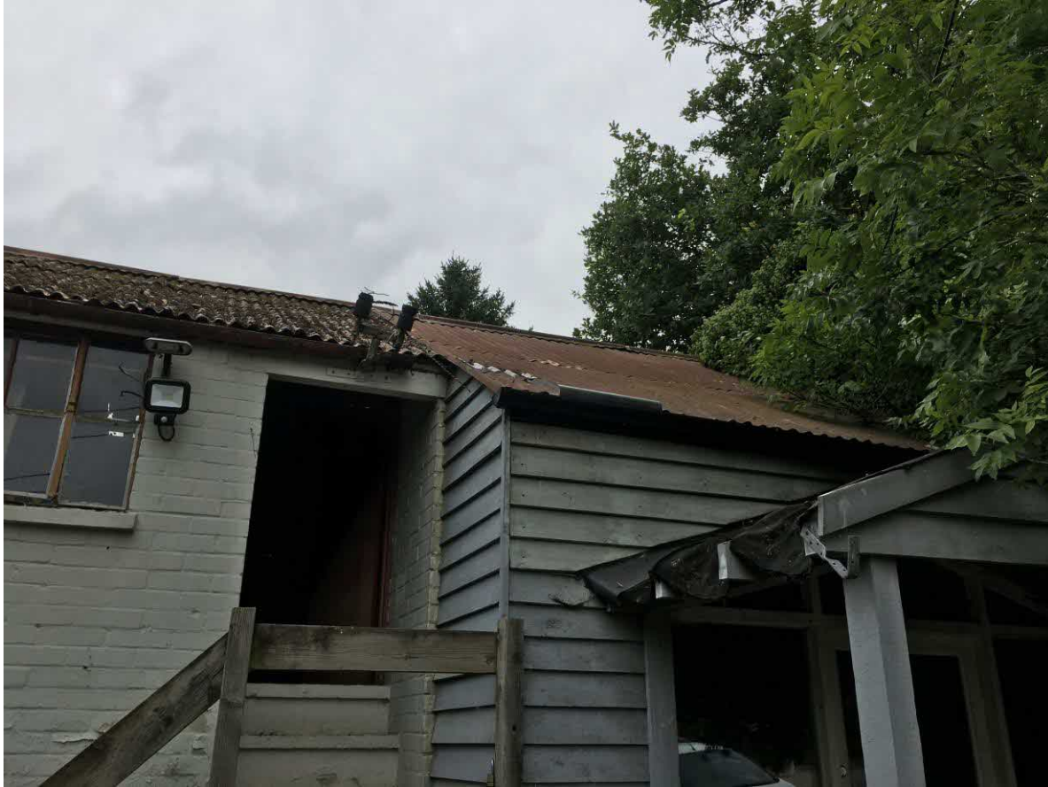
Asbestos roof panels
