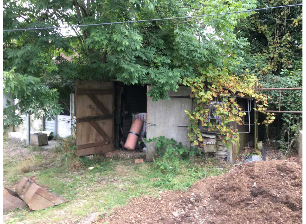
Shed on adjoining land
