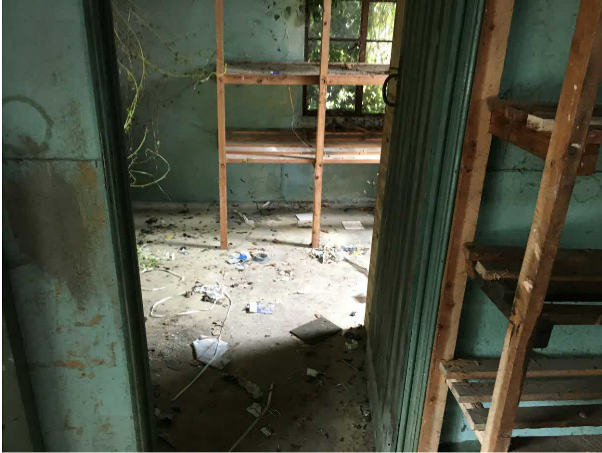
First floor storage
