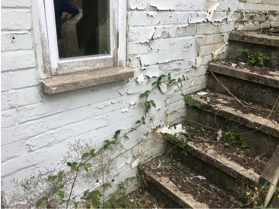
Stairs to first floor
