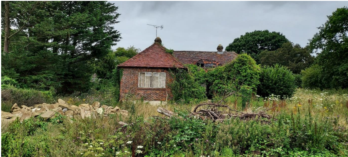
Photo 5: One-storey dwelling near the centre of the site (building 5)
