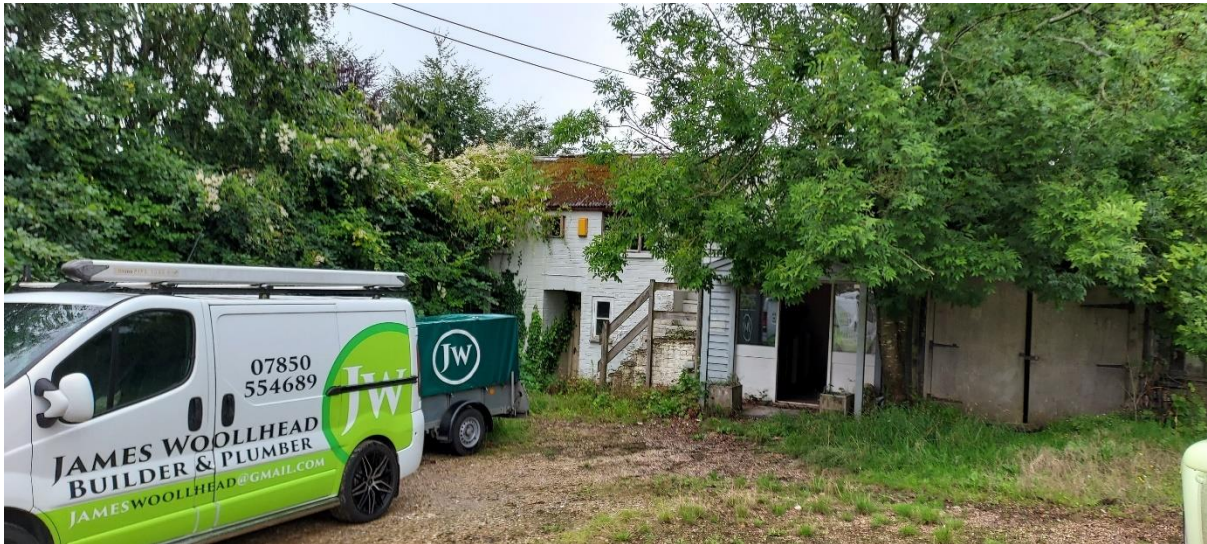
Photo 1: Office building in south-west corner (building 1)
