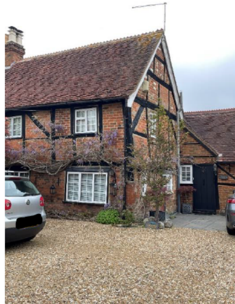
Main entrance to the building
