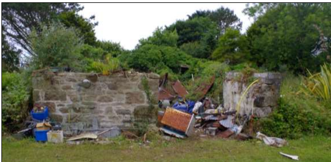
FIGURE 12: THE NORTH-EAST ELEVATION OF THE BARN; VIEWED FROM THE NORTH-EAST (1M SCALE).
