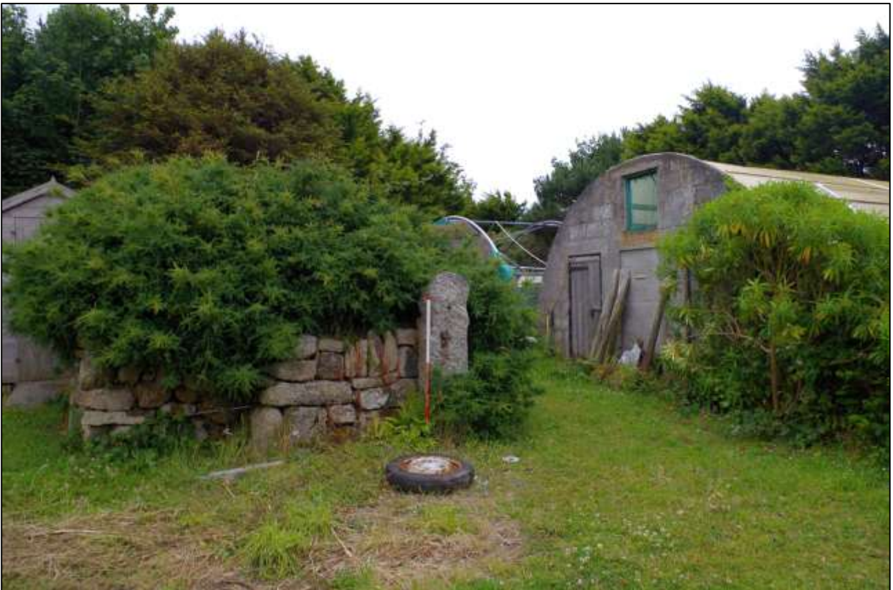
2. THE MODERN GARDEN BUILDINGS TO THE SOUTH-EAST, WITH (REUSED) GRANITE GATEPOST AND LATER GARDEN WALLS; VIEWED FROM THE NORTH-WEST (1M SCALE).
