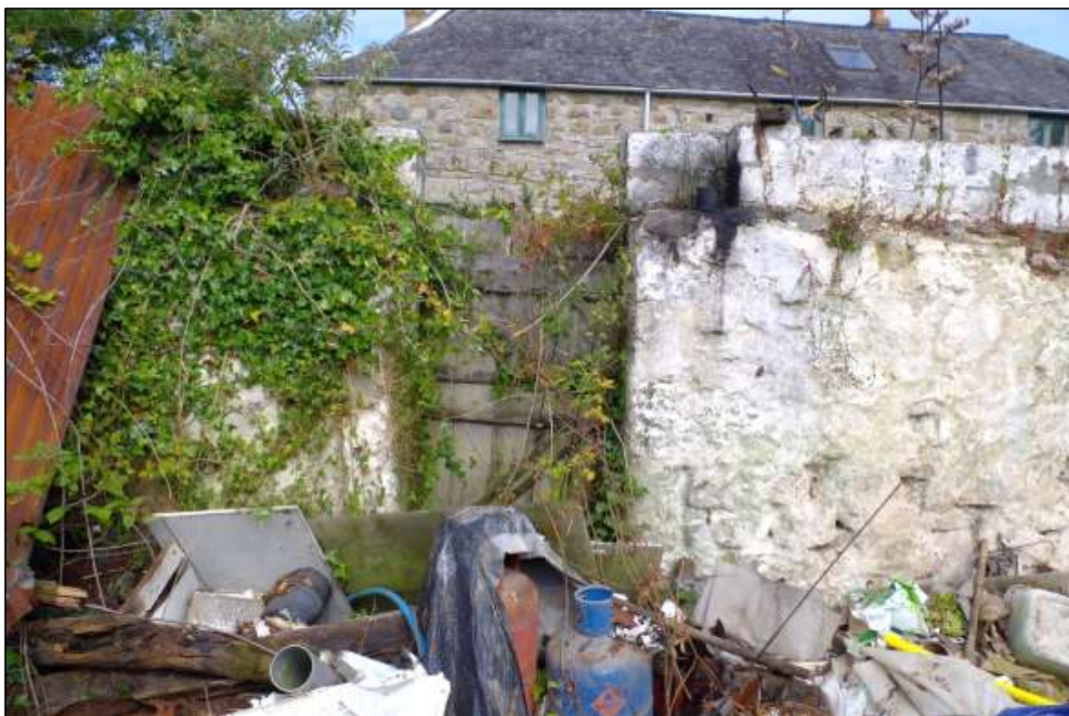
FIGURE 16: A DOOR OPENING IN THE NORTH-WEST ELEVATION; VIEWED FROM THE SOUTH-EAST.
