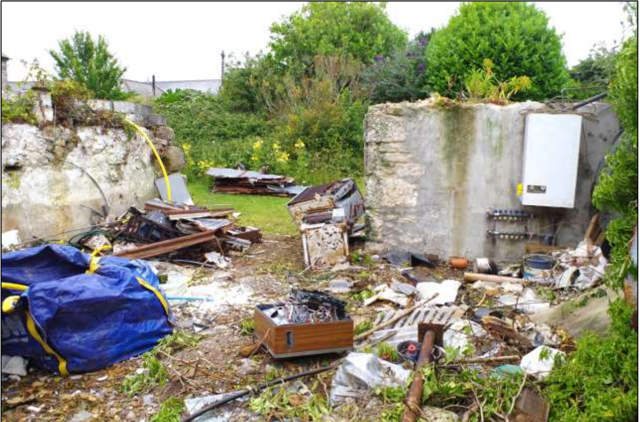
7. THE INTERNAL NORTH-EASTERN ELEVATION; VIEWED FROM THE SOUTH.
