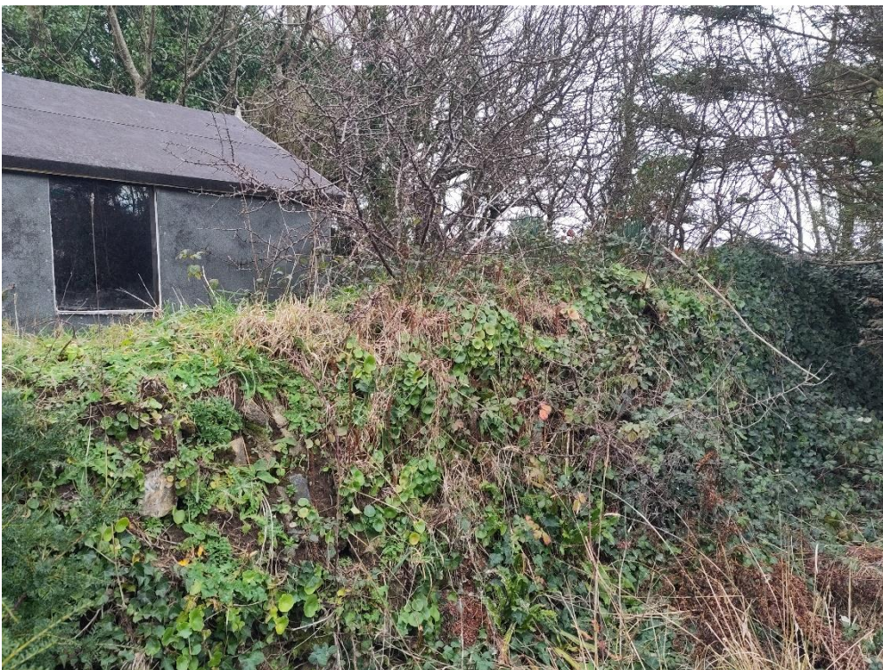
Photo 19: H3 adjacent to the shed.
