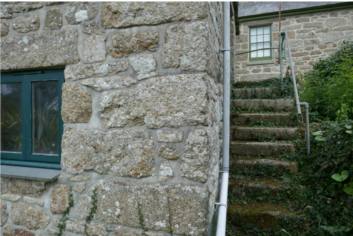
Figure 3. Flight of stone steps on the north side of the granary.
