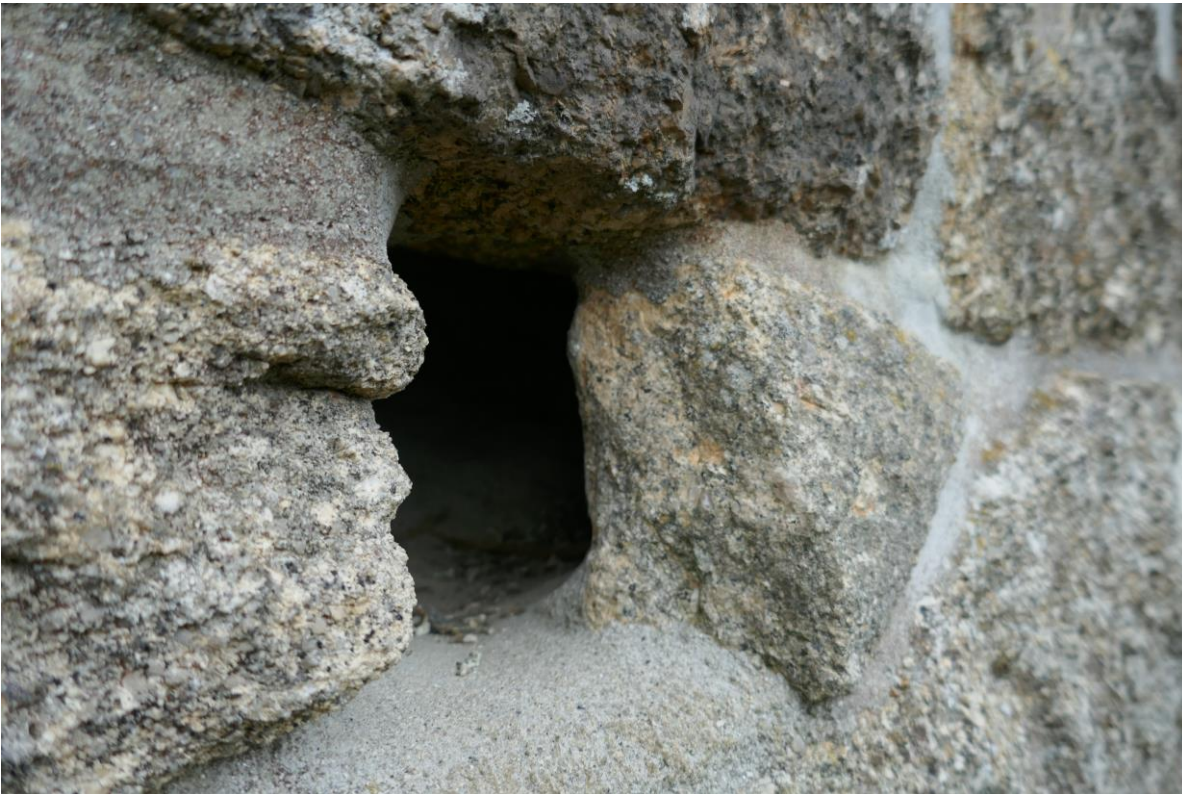
Figure 2. Close-up of one of the square holes in the eastern aspect of the building.
