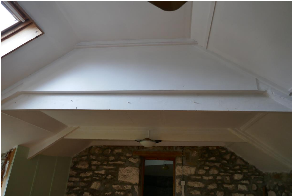
Figure 6. Boxed void on the upper floor of the granary.
