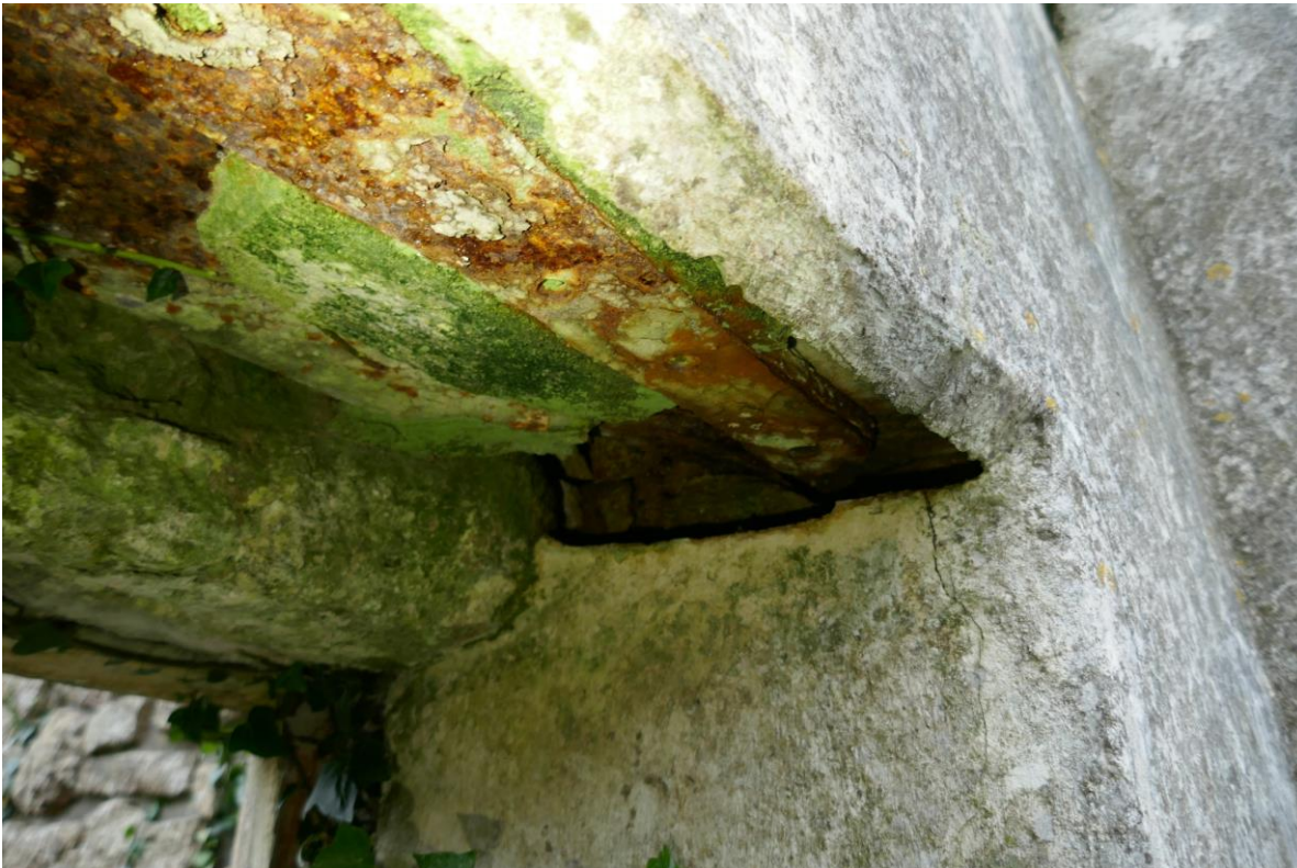
Figure 9. Recess leading into the stonework at the edge of the lean-to entrance.
