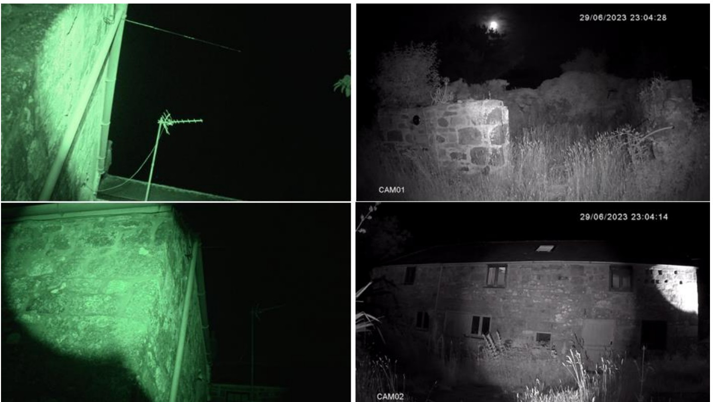
Figure 3. Infrared illumination. Top left: IR Surveyor, Granary northern aspect, 11 May 2023. Top right: Surveyor 2, Collapsed barn, 29 June 2023. Bottom left: IR Surveyor, Granary northern aspect, 29 June 2023. Bottom right: Surveyor 2, Granary eastern aspect, 29 June 2023.
