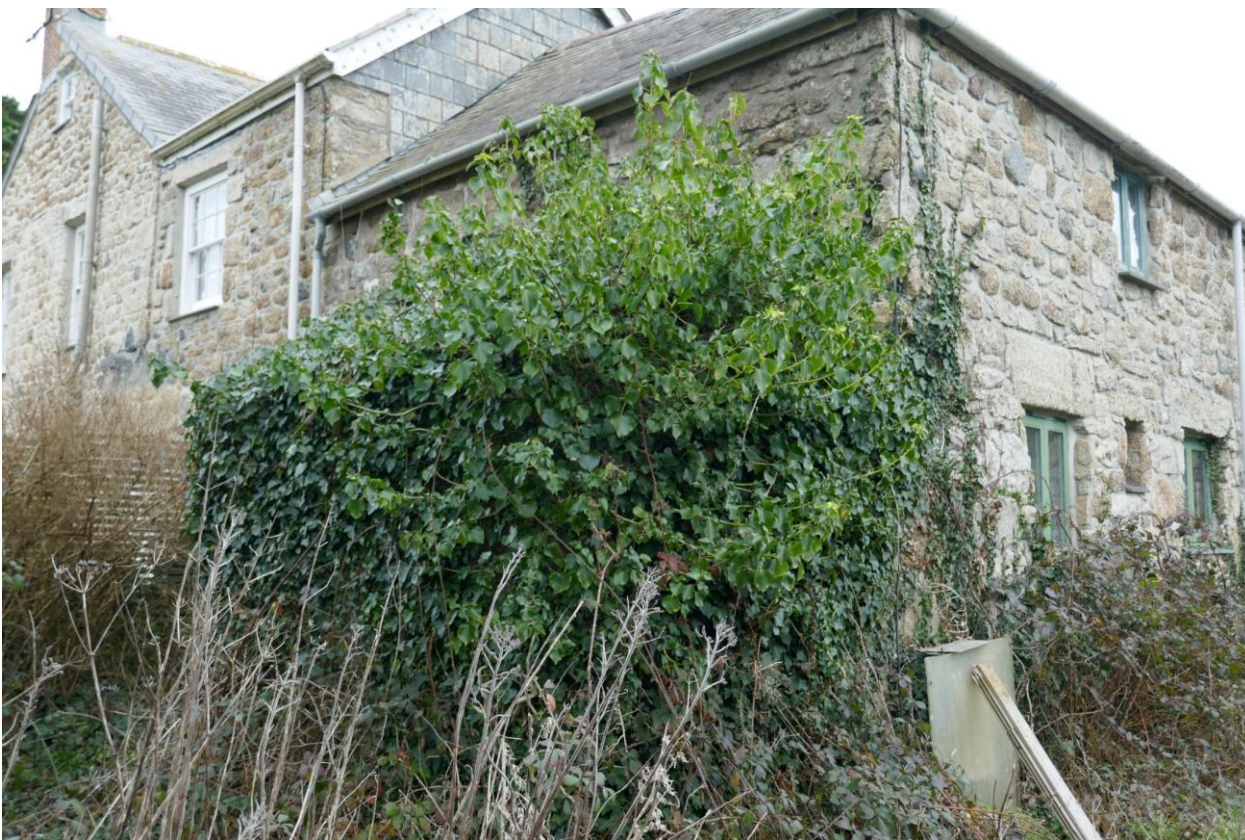
Figure 7. Ivy-covered lean-to on the south side of the granary.
