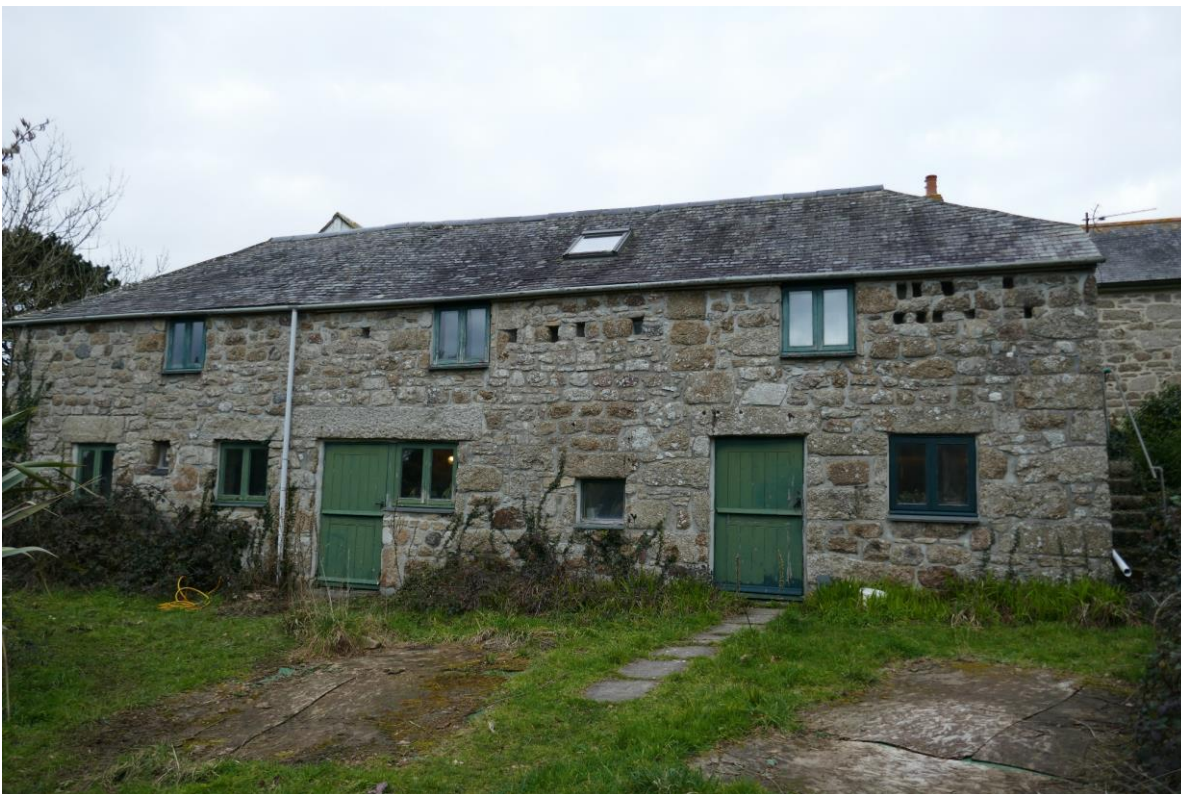
Figure 1. Eastern aspect of the granary.
