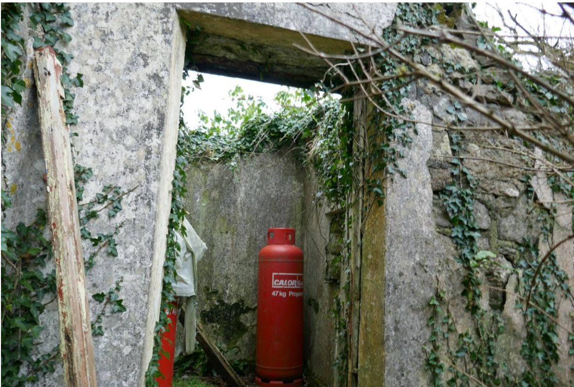
Figure 8. Entrance to the lean-to on the west side.
