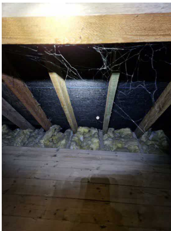
Plate 8: A photograph of the floor insulation, plyboard flooring installation and bitumen felt in the roof void.
