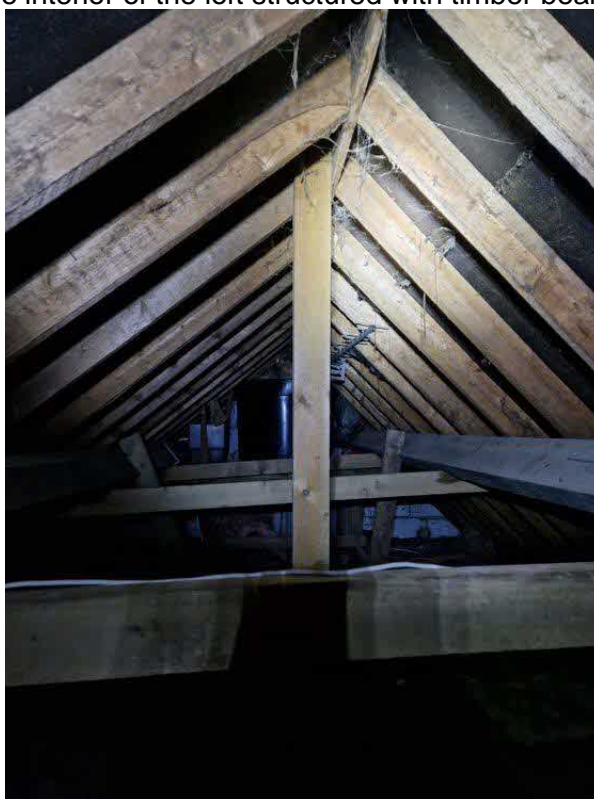
Plate 6: Evidence of the interior of the loft structured with timber beam.
