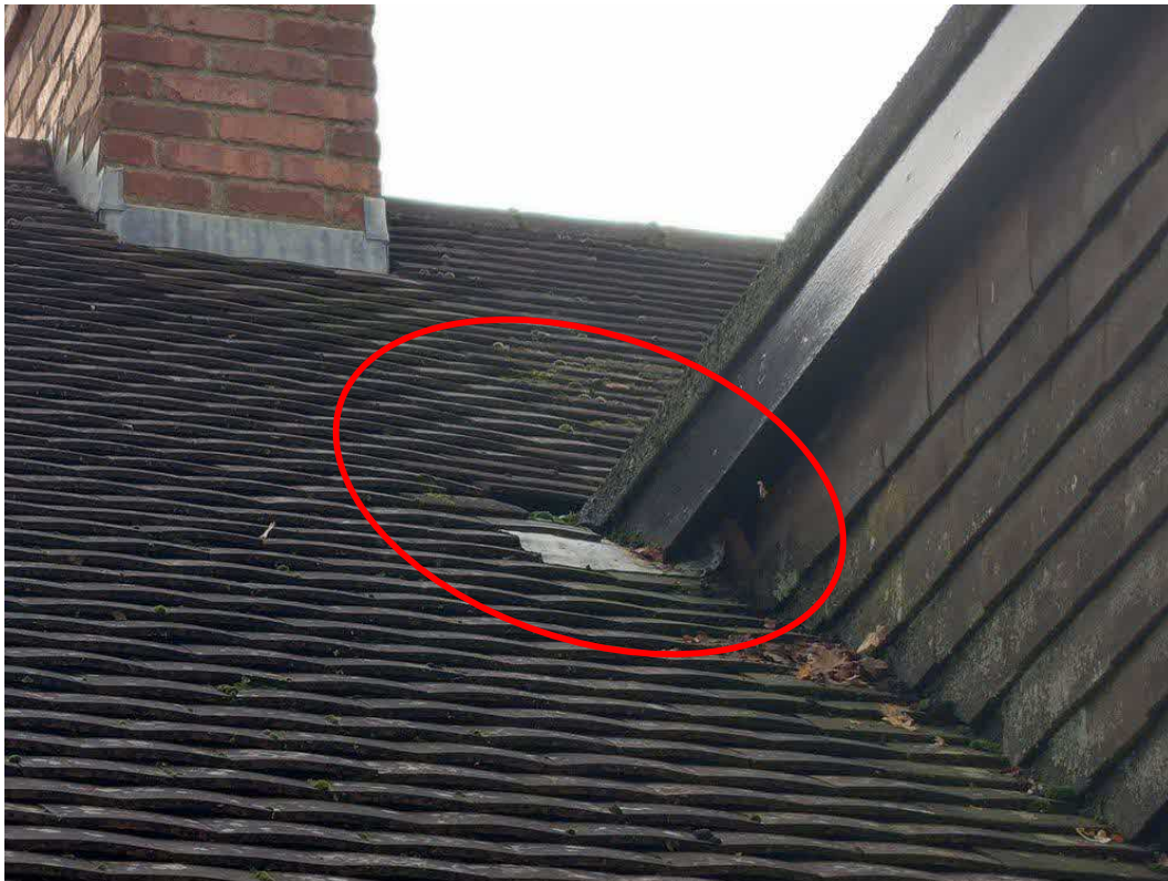
Plate 4: Evidence of a ridge gap on the southern elevation.
