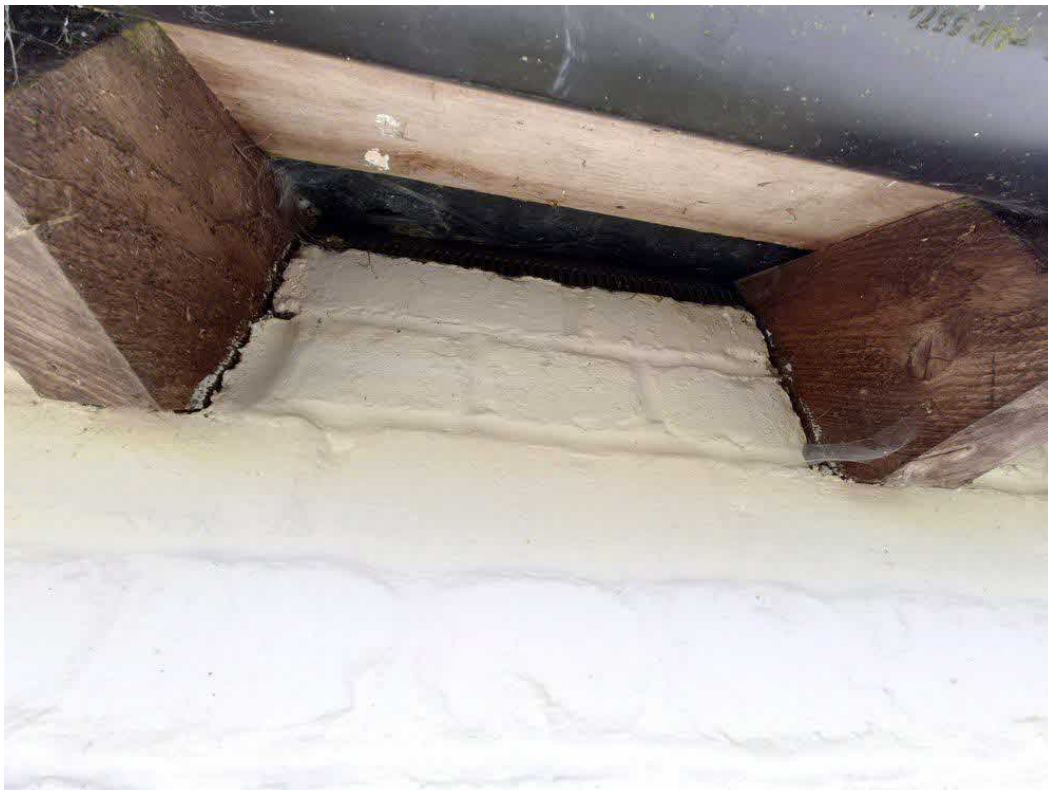
Plate 10: Evidence of venting in the north elevation of the building.
