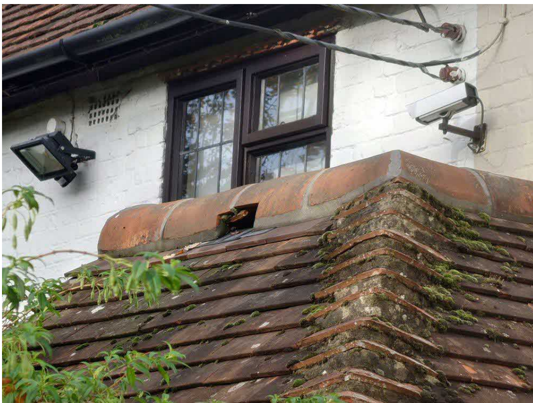
Plate 4: Evidence of a ridge gap on the southern elevation.
