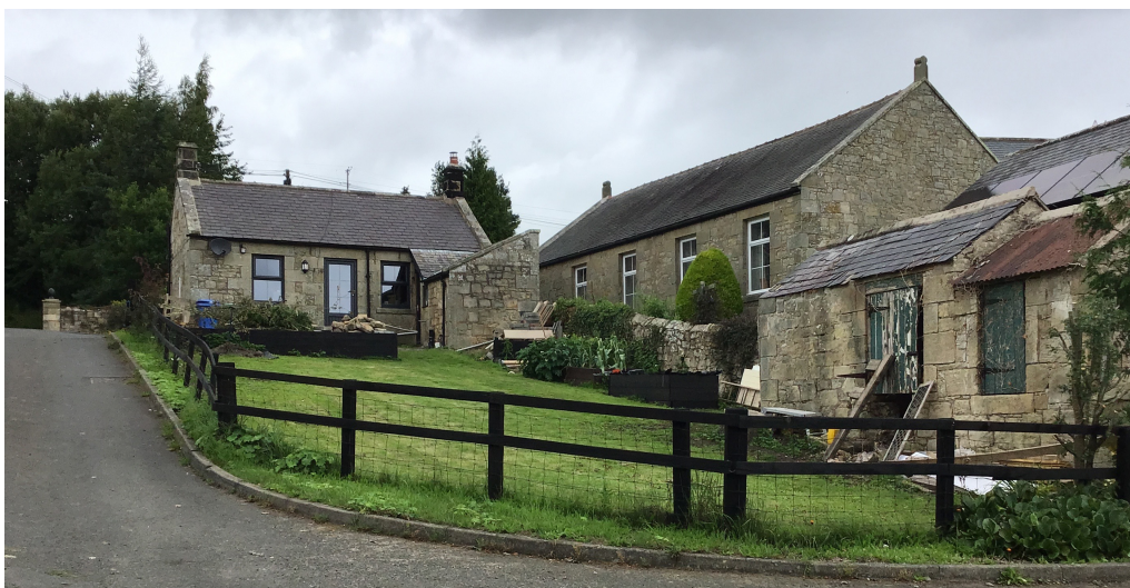
View of No15 West Turnpike from the south
