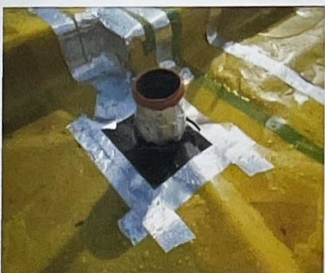
Photograph 4: Check top hat is sealed to membrane and pipework. If the formed top hat is not tight to the pipework, then also confirm presence of jubilee clip beneath butyl tape.
