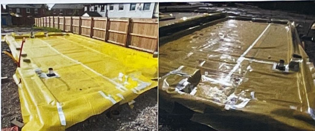
Photographs 1 and 2: Check general condition of membrane for punctures / tears etc
