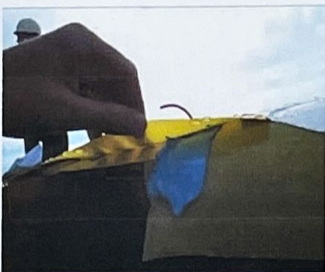
Photographs 1 and 2: Check general condition of membrane for punctures / tears etc
