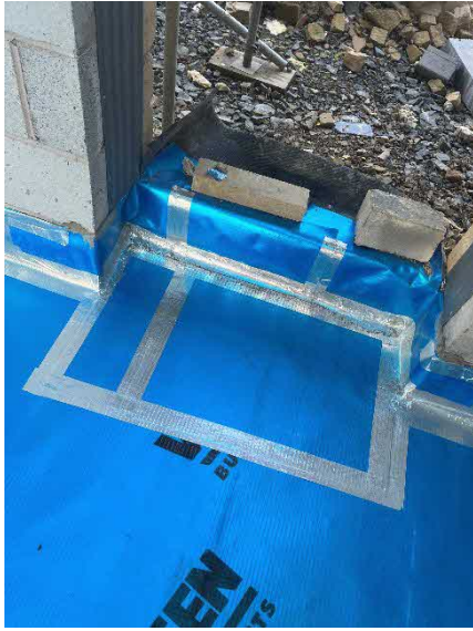
General condition of membrane of corner units and joints within the garage plot.
