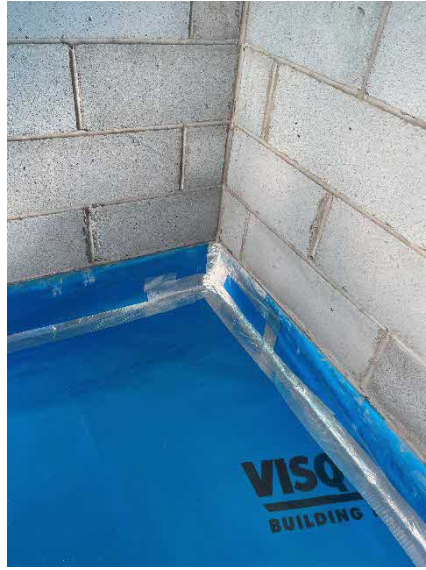
General condition of membrane of corner units and joints within the garage plot.
