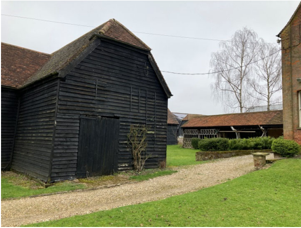
South Elevation of Barn K (Hixham Hall to the right and Barn I in the centre)
