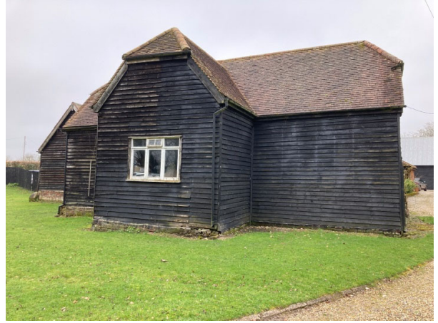
West Elevation of Barn K (Barn J behind on the left)
