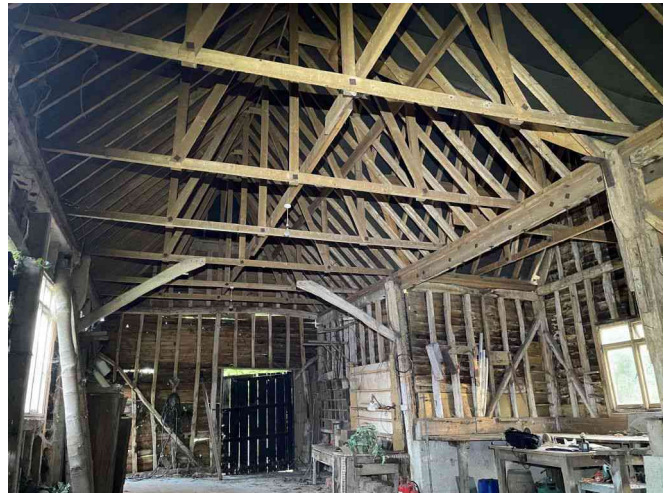
Photograph 4: Internal view of Barn K.
