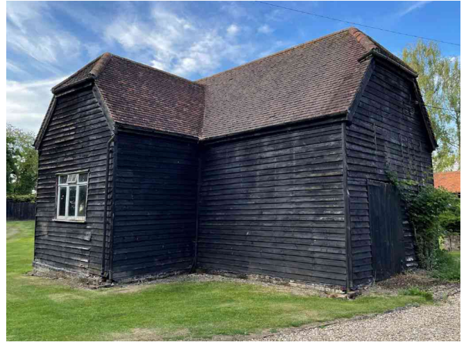
Photograph 2: West and south gable ends of Barn K.
