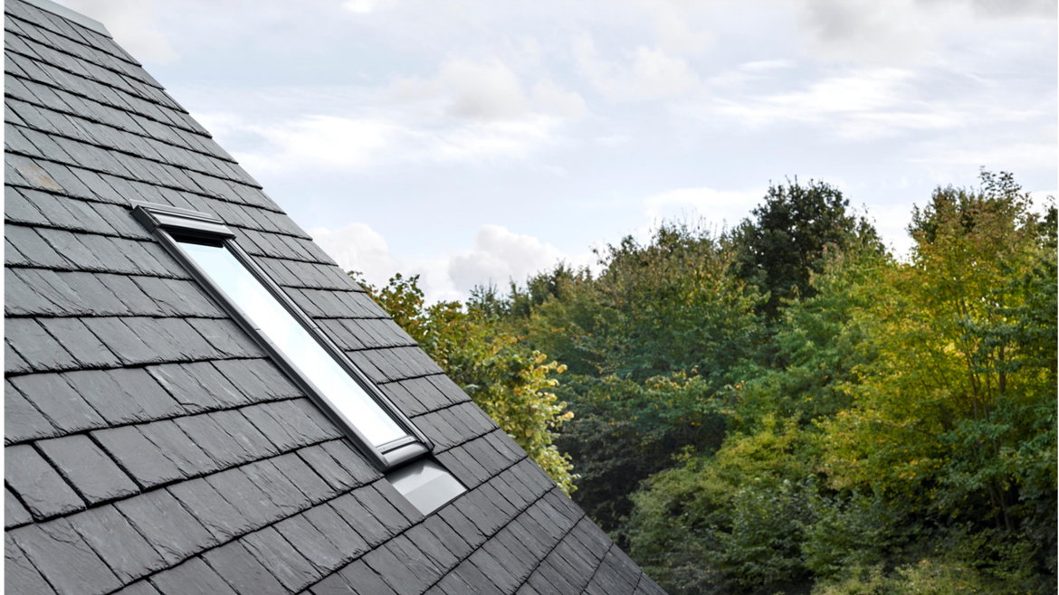
Example of Velux rooflight in recessed slate flashing kit
