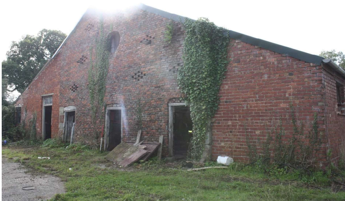
Plate 9 North elevation of the barn, facing southeast.
