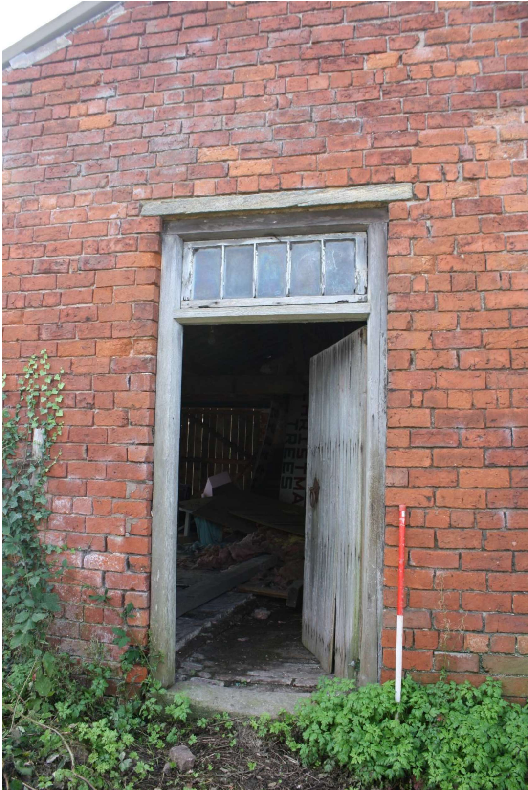
Plate 10 Door with transom window in the east outshut.
