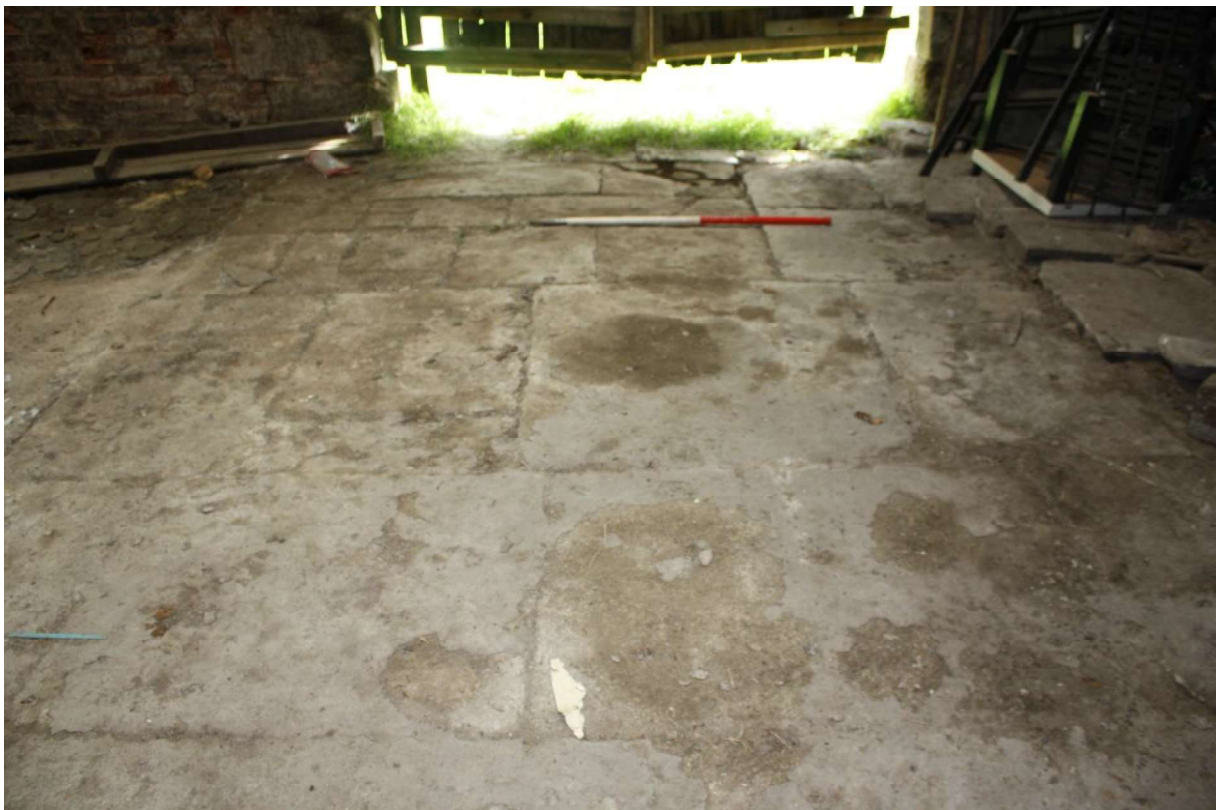
Plate 18 Flagged threshing floor, facing east.
