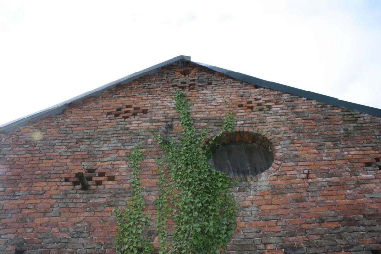
Plate 12 North elevation with a pitching eye and ventilation slots.
