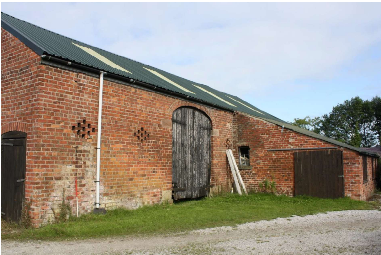
Plate 3 East elevation of the barn, facing northwest.
