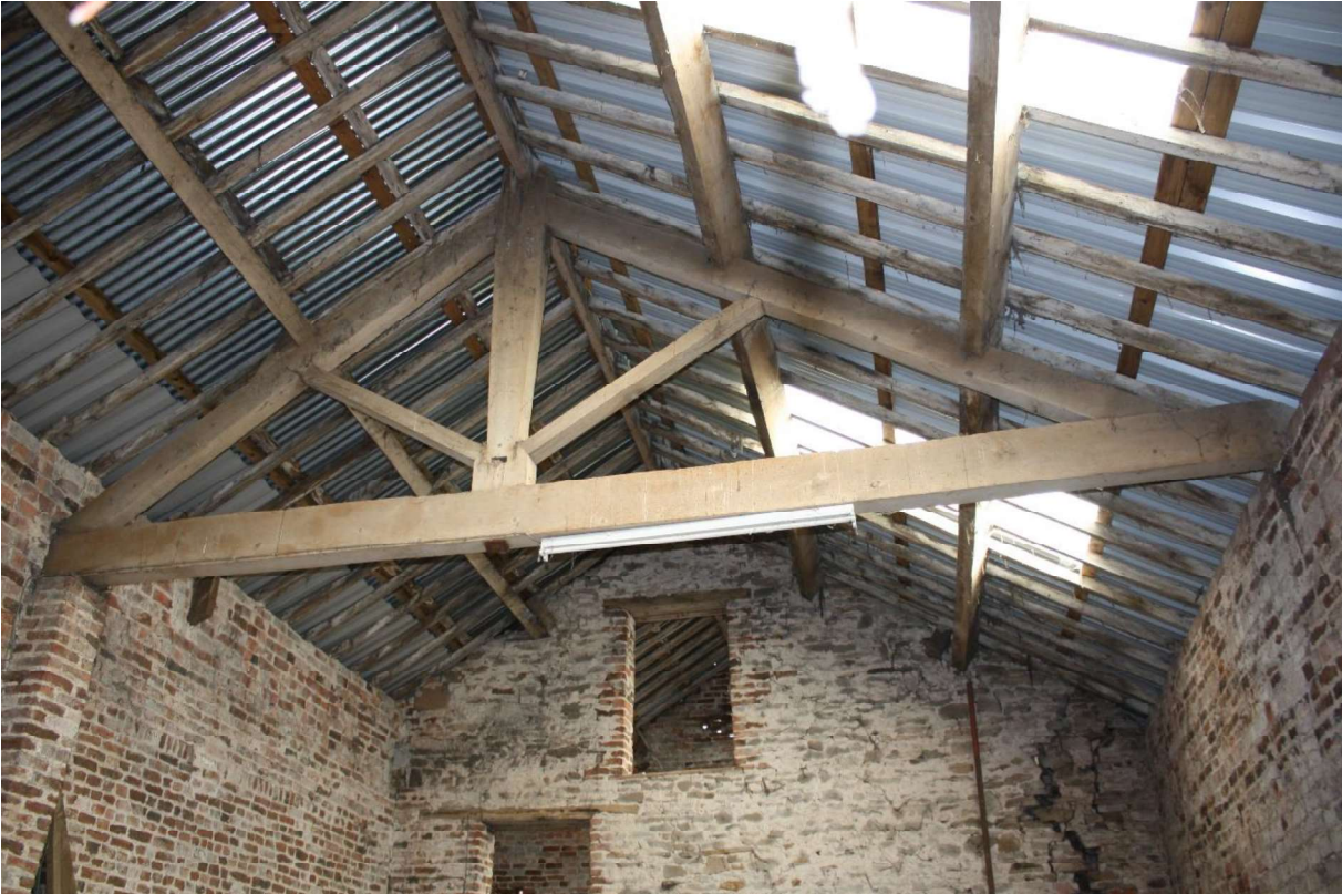
Plate 20 King post truss supported on a brick pillar.
