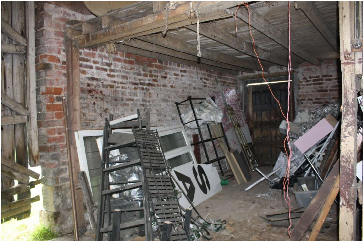
Plate 27 Storage room under a south hayloft, facing southwest.
