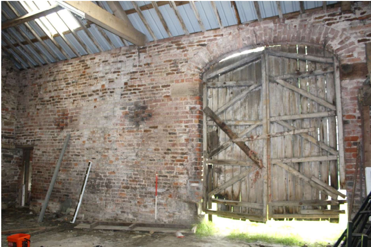
Plate 17 East internal elevation with wagon door, facing northeast.
