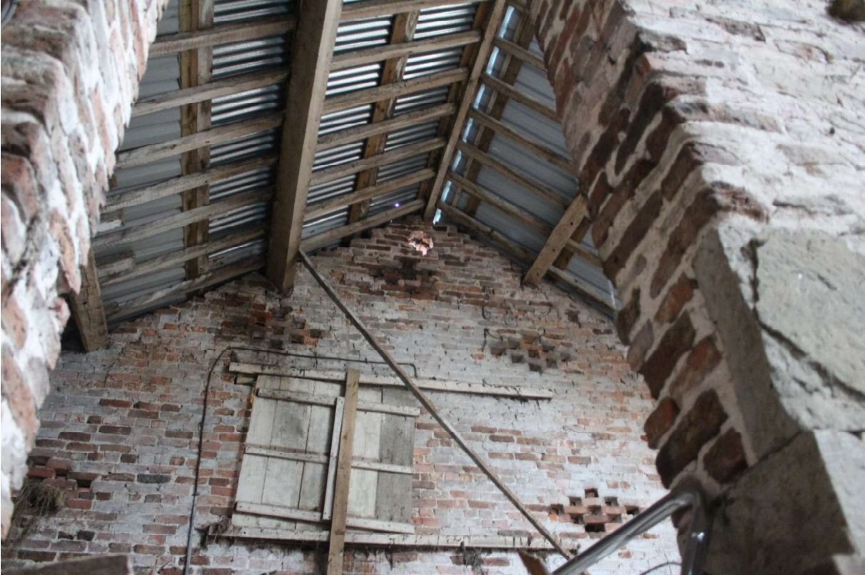
Plate 16 North gable with sliding pitching door.
