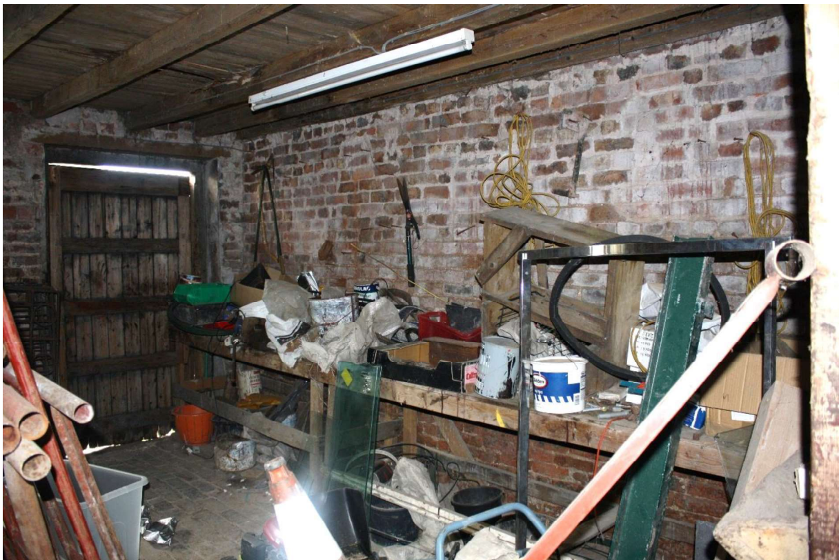
Plate 28 Storage room under a south hayloft, facing southeast.
