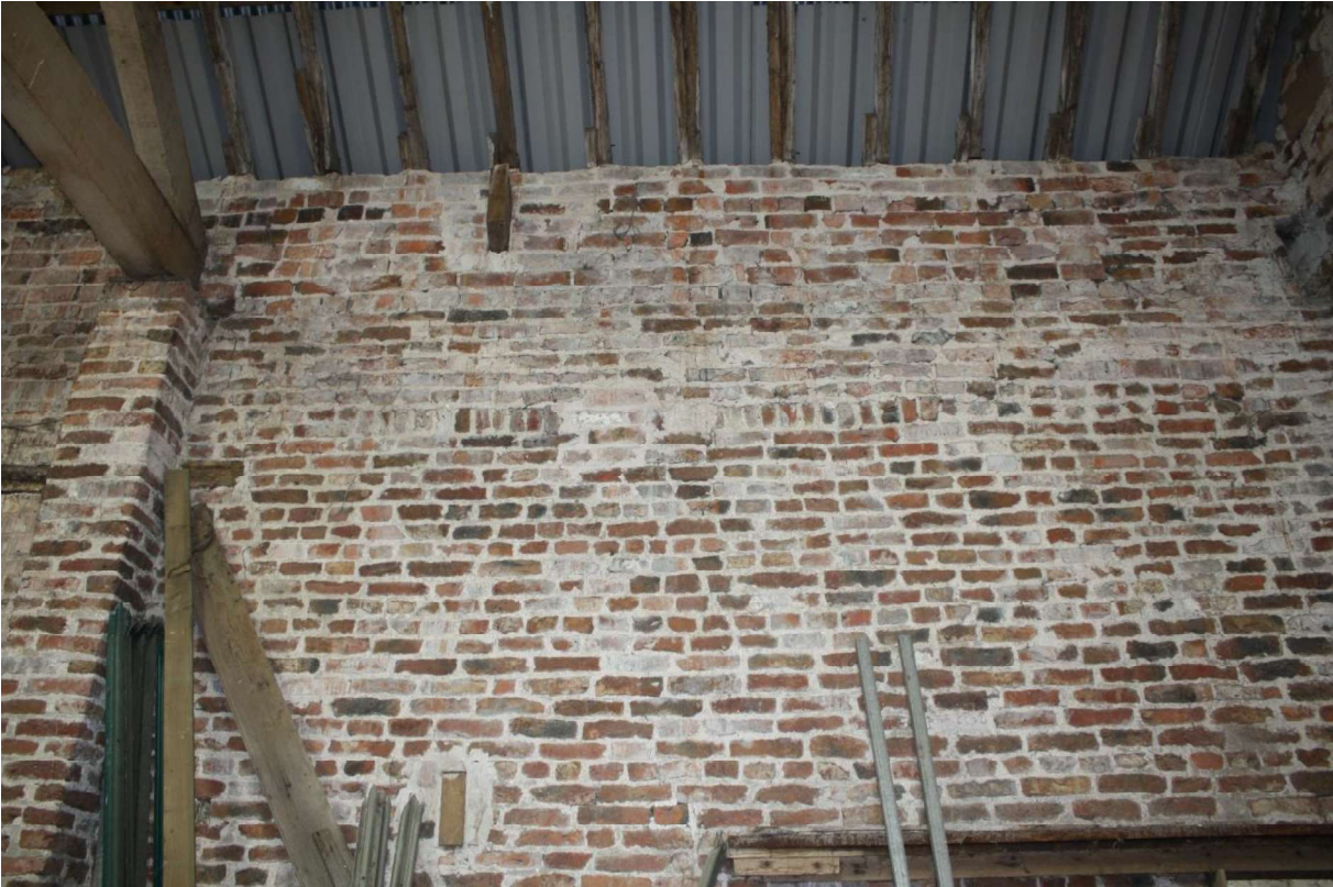
Plate 25 Fragment of west internal elevation with two lines of rowlock course inserted.
