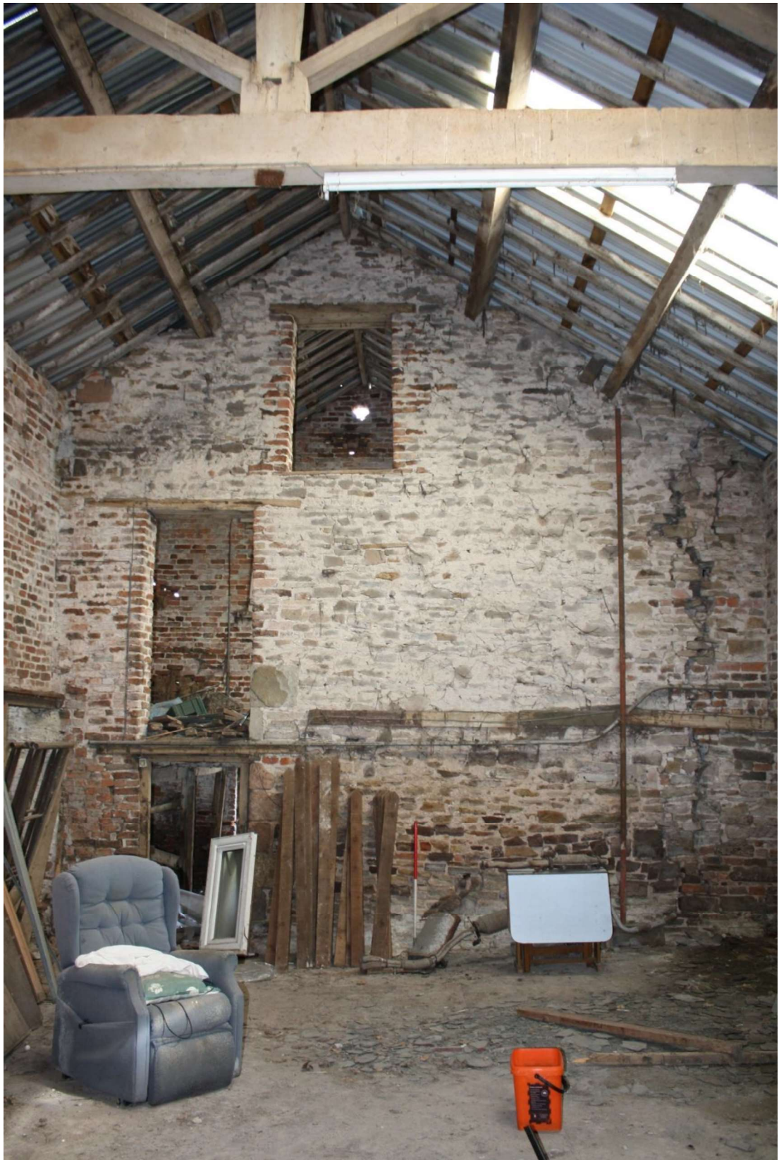
Plate 15 Partition wall in the main range, facing north.
