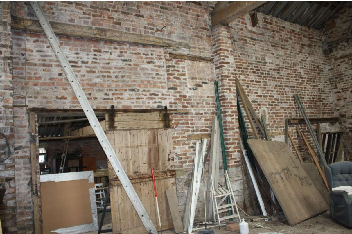
Plate 23 West internal elevation facing northwest.
