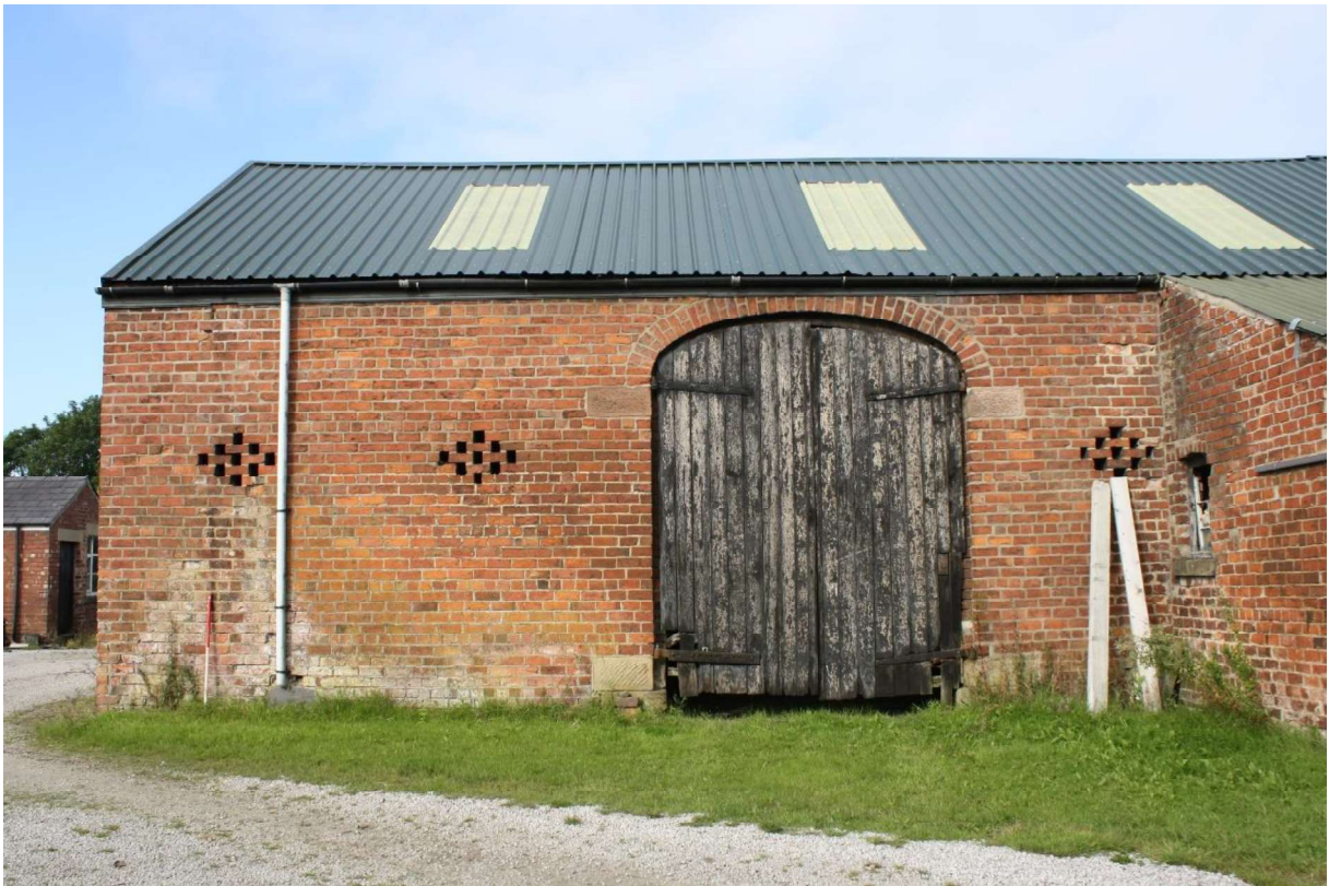
Plate 4 South part of the east elevation, facing west. The large wagon door displays the evidence of lowering of the roof.
