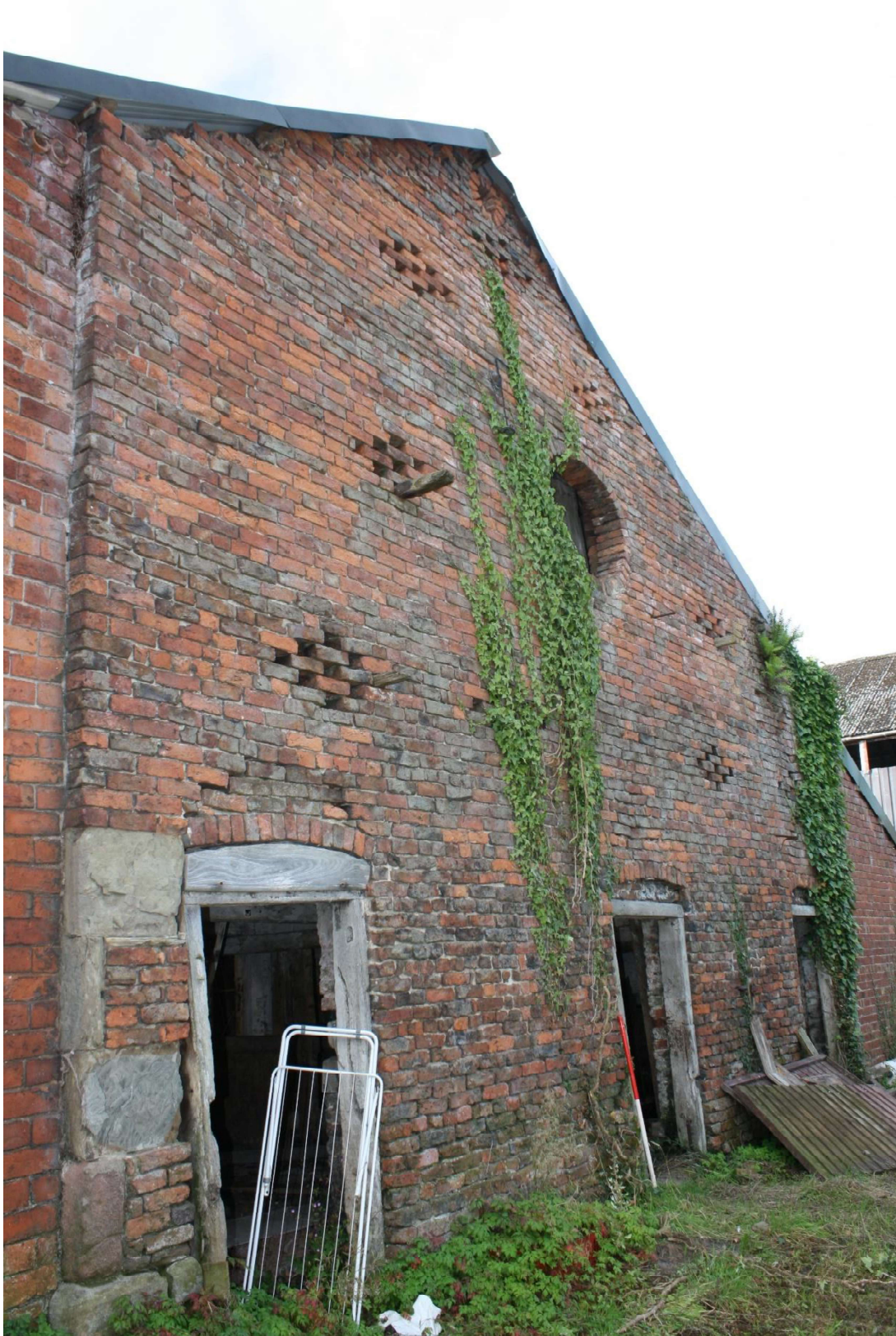
Plate 11 North elevation of the barn, facing southwest.
