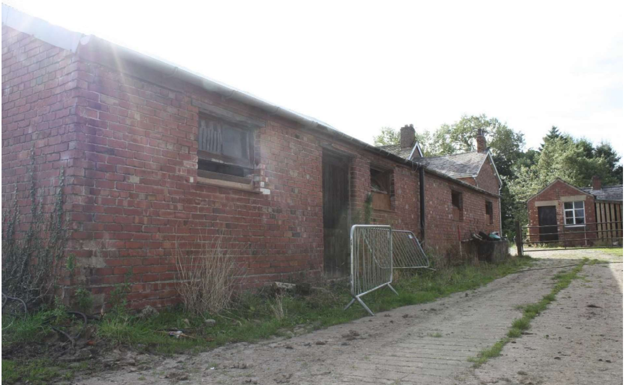
Plate 7 West elevation of the barn, facing southeast.
