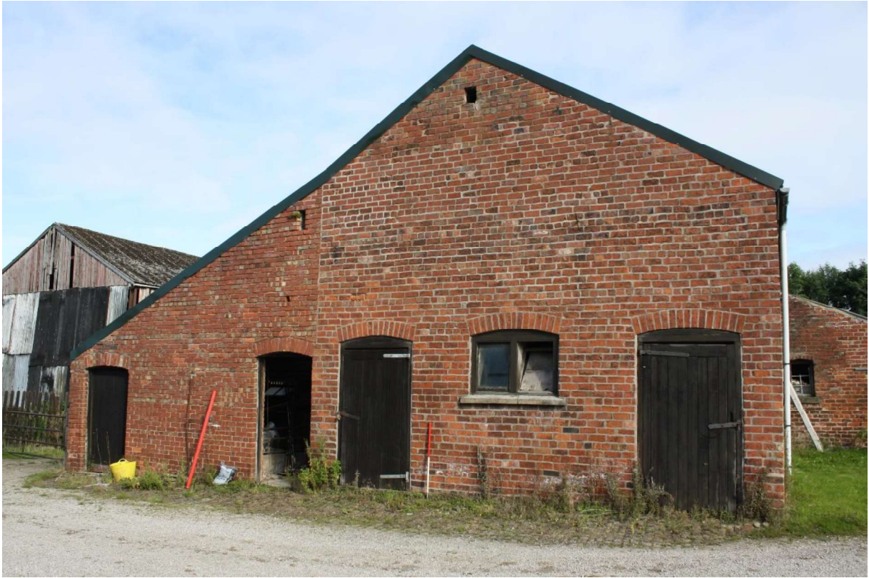
Plate 1 South elevation of the barn, facing northwest.
