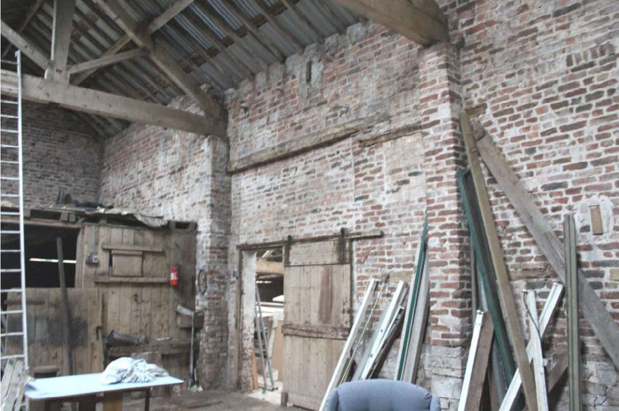
Plate 22 West internal elevation, facing southwest.
