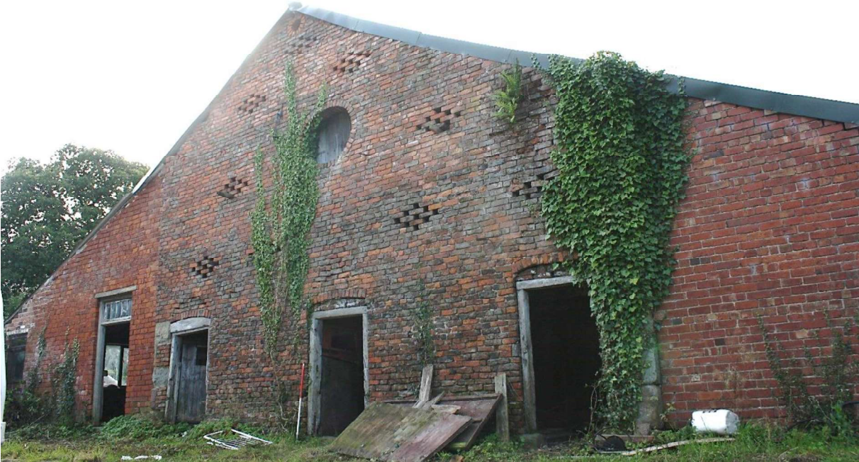
Plate 13 North elevation of the barn, facing southeast.
