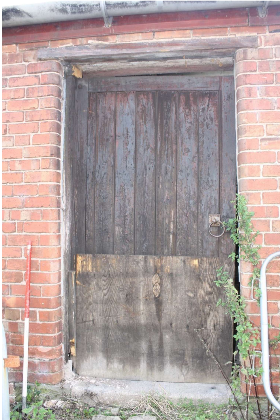
Plate 8 West outshut door, facing east.
