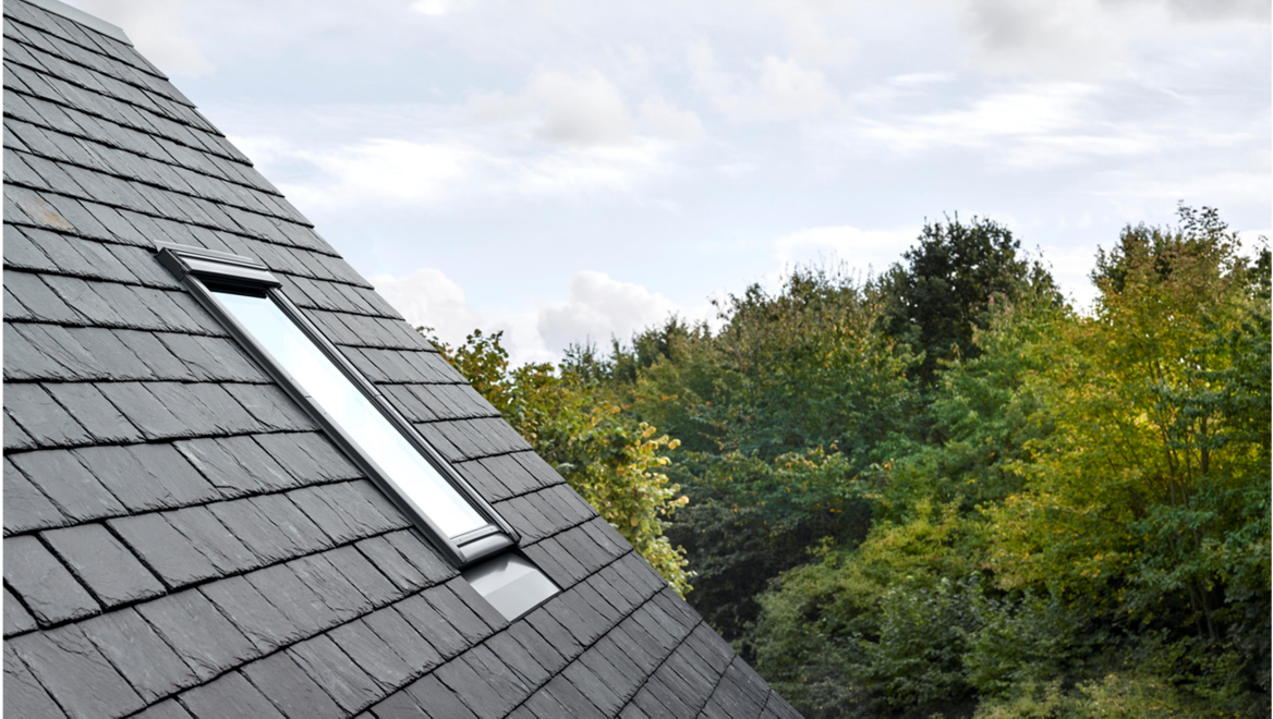
Example of Velux rooflight in recessed slate flashing kit
