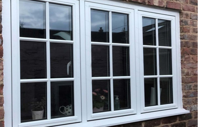
Example of pre-finished engineered timber windows with glazing bars
