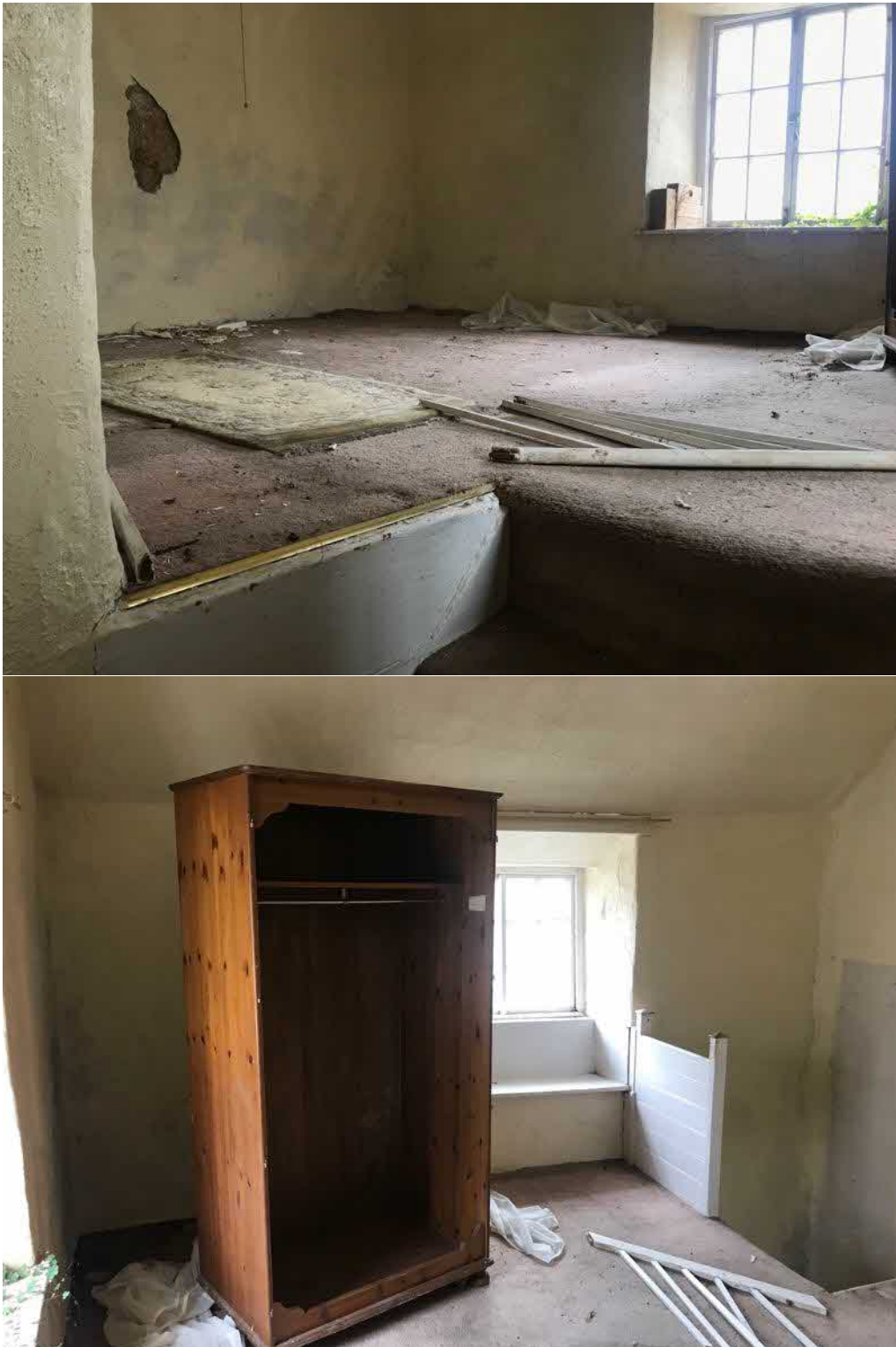
Figure 12: Views of the southeast and north sides of the main room, first floor
