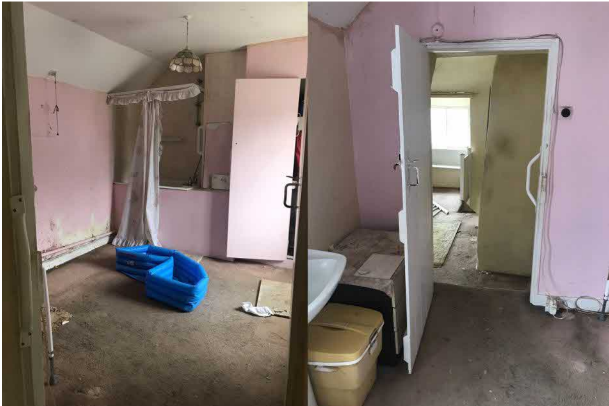
Figure 16: Composite view looking east and west into the kitchen wing
