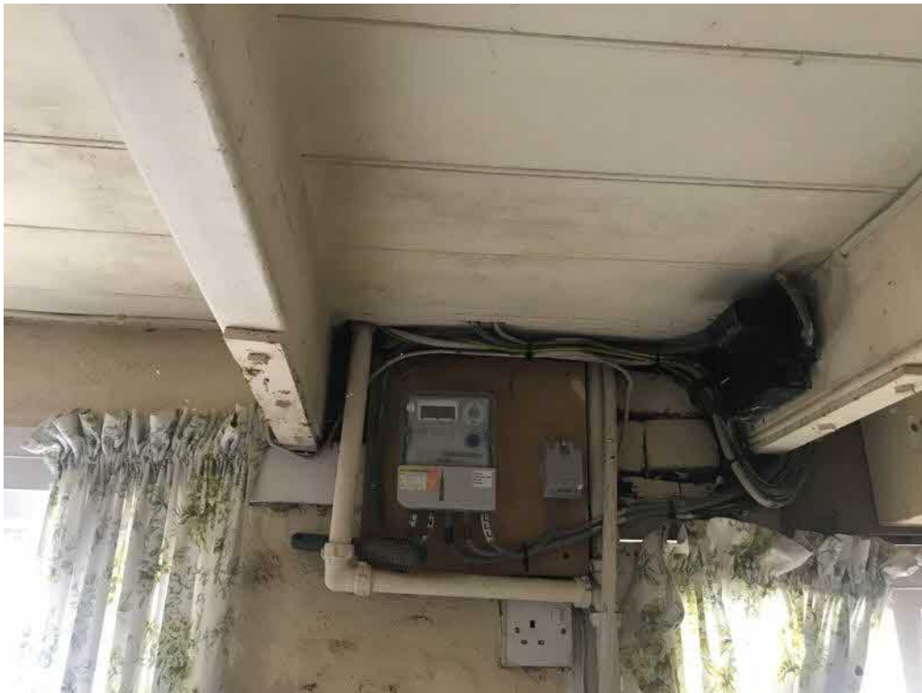
Figure 10: Detail of ad hoc pipework and brickwork in south wall.
