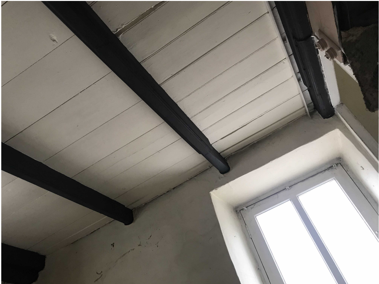
Figure 8: Detail of floor joists, seen from ground floor main room
