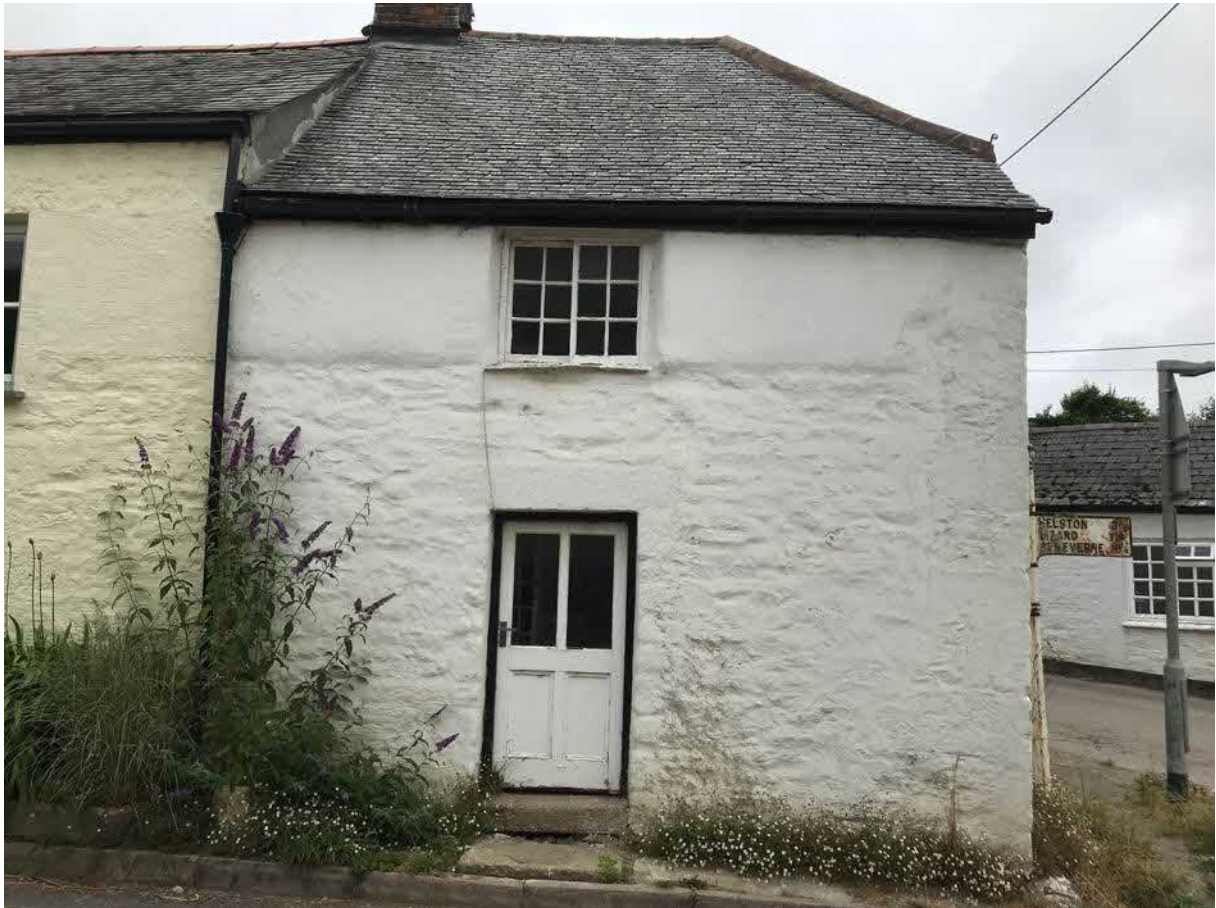
Figure 3: West elevation of Alpha Cottage, showing construction techniques
