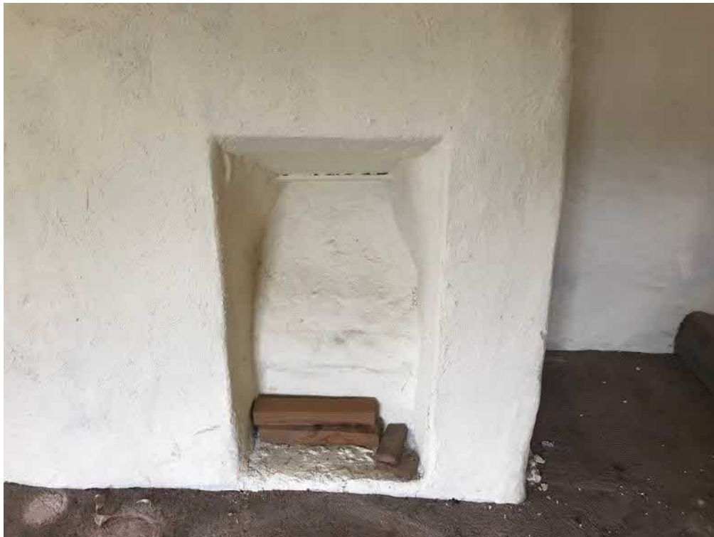
Figure 13: Detail of chimney breast on the first floor.
