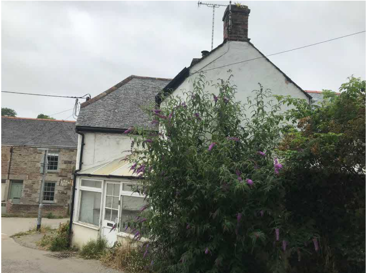
Figure 4: East elevation of Alpha Cottage
