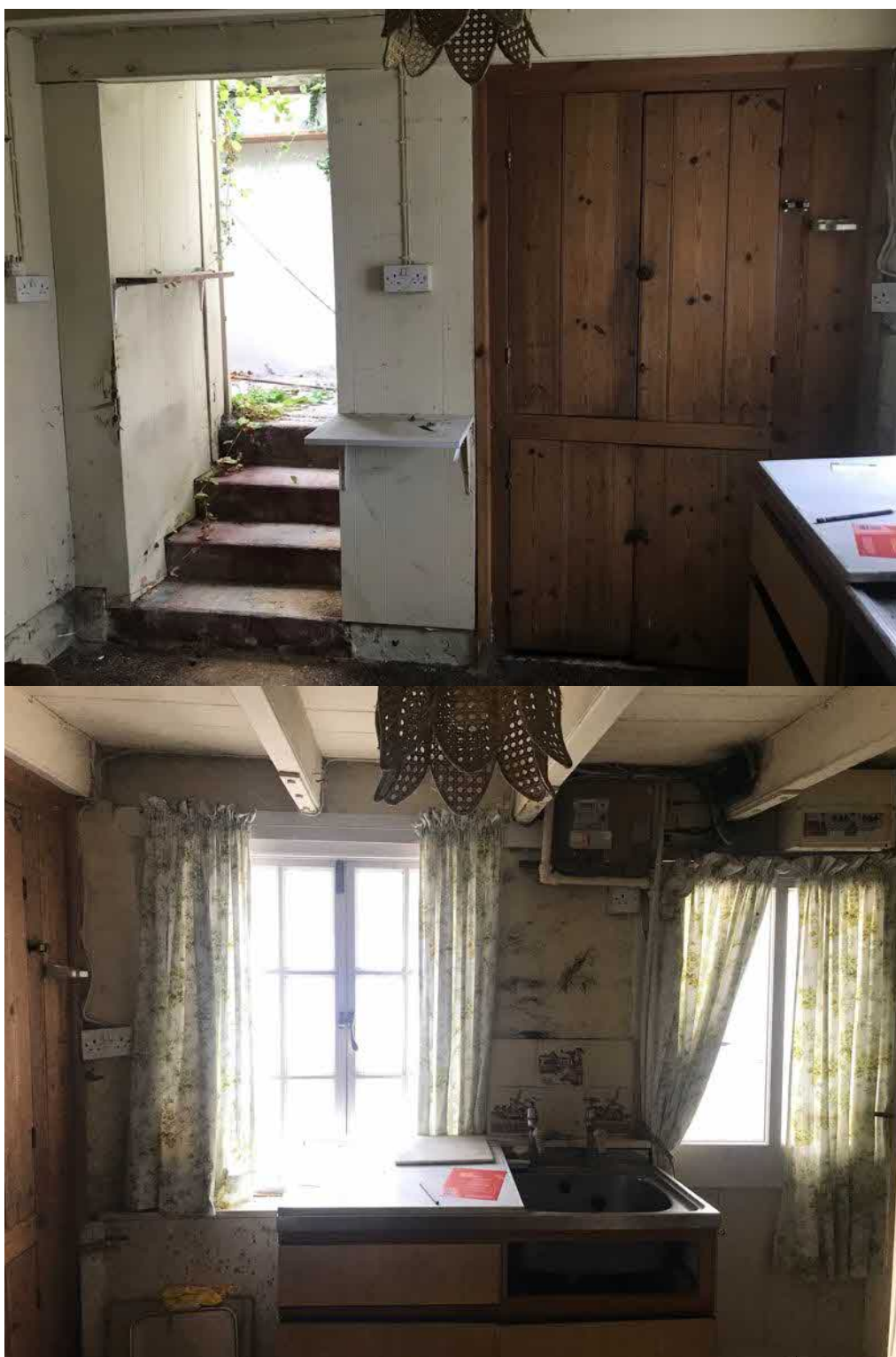
Figure 11: East and south walls of the kitchen wing
