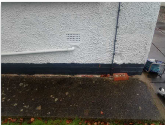
Fig 11: Trial Hole 1 Location
