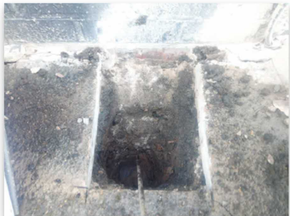
Fig 12: Trial Hole 1 Footing
