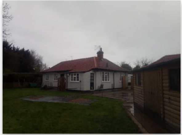
Fig 3.2: Rear of property
