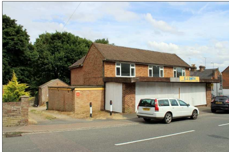
Plate 5: Side and front elevations, facing southeast
