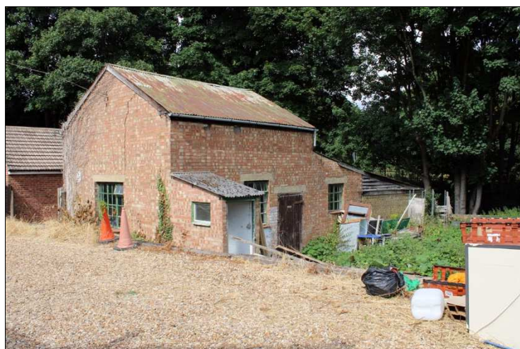
Plate 10: Brick outbuilding, facing north-northeast
