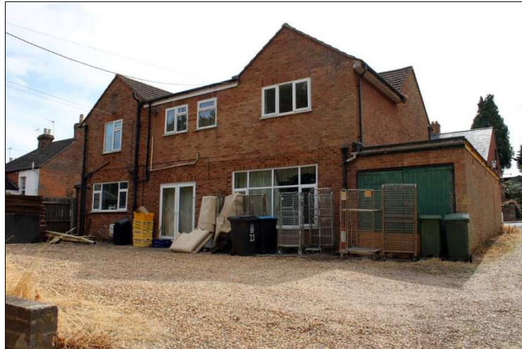
Plate 7: Rear elevation, facing southwest
