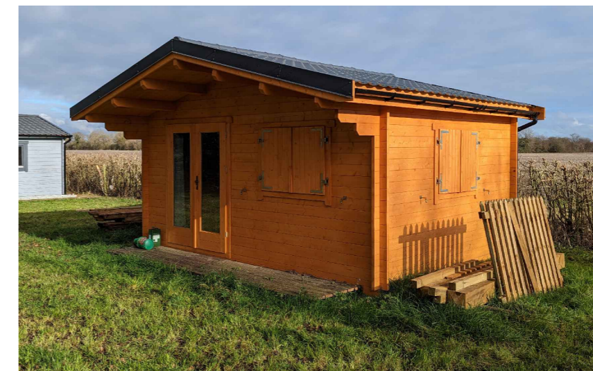
South West/South East Elevation - Photo - NTS (Unit 1)
