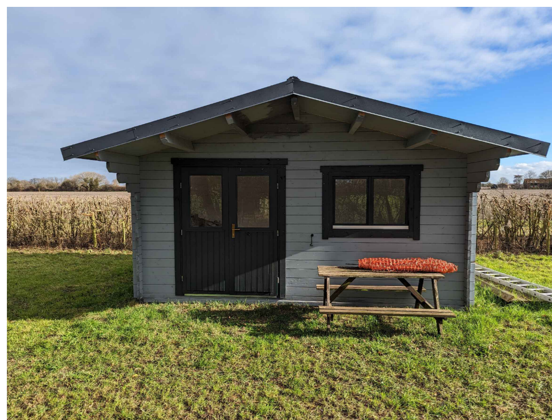
South West Elevation - Photo - NTS (Unit 2)
