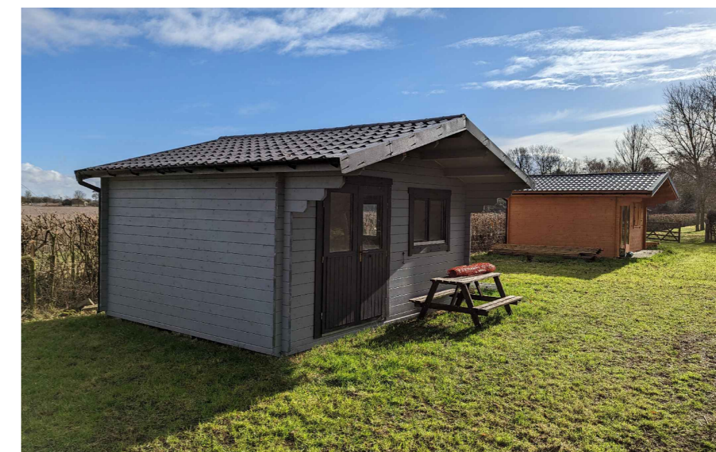
North West/South West Elevation - Photo - NTS (Unit 2/1)
