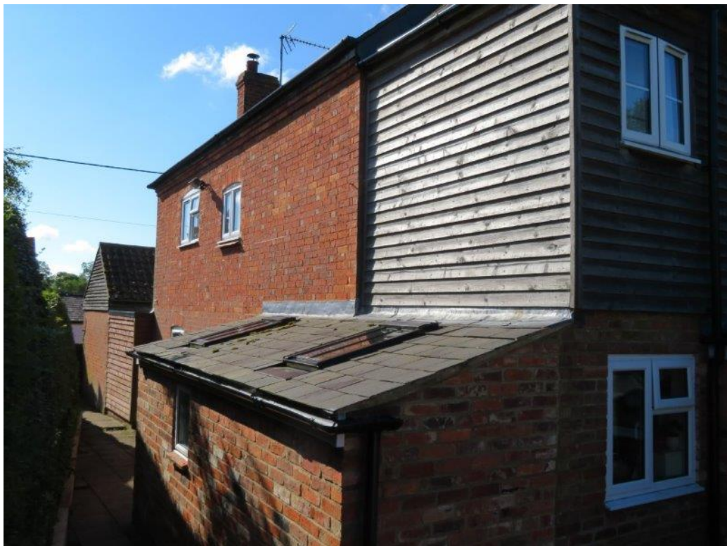
Part Rear view of house
