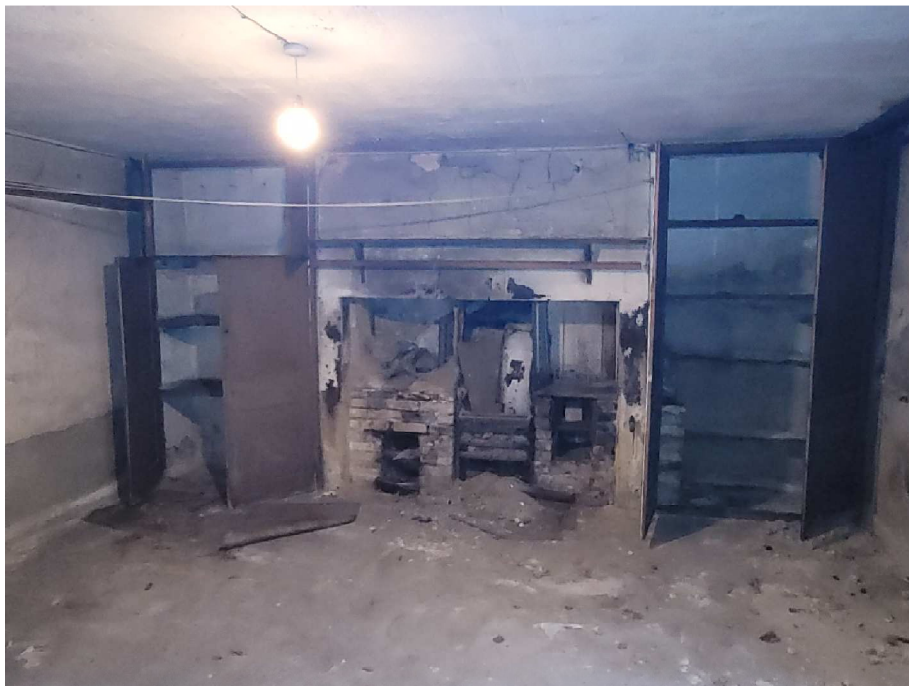
Fireplace to proposed cinema room. Wood burning stove to be fitted
