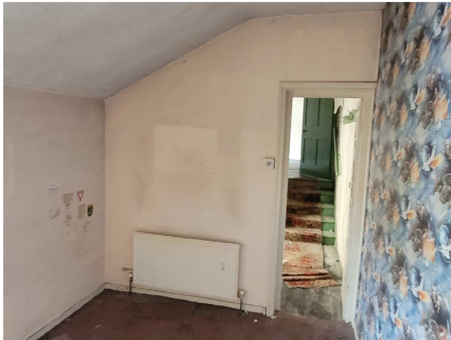
First floor lower rear addition. Remove wall and form master ensuite and dressing room.
