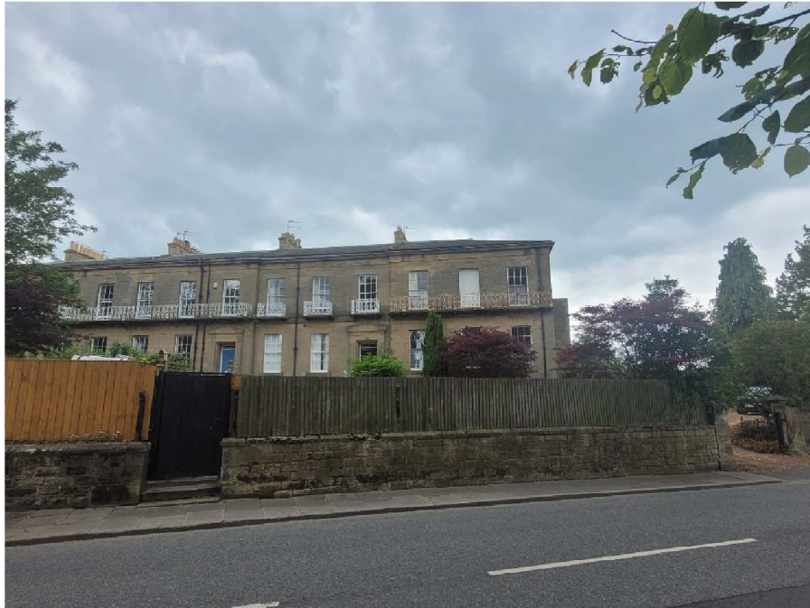
Existing front elevation from South Road
