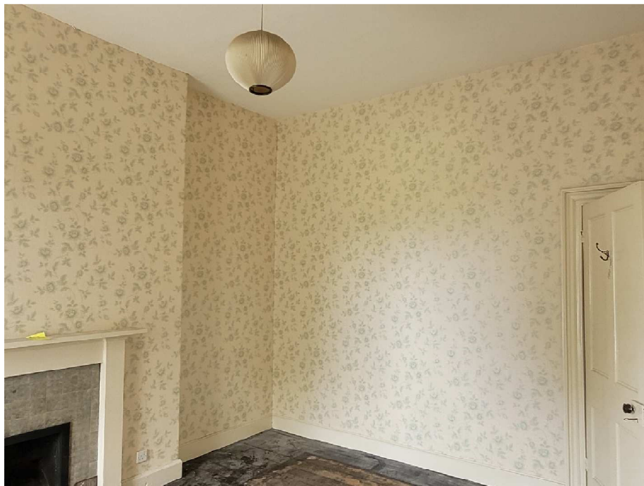
Bedroom 2. Remove section of wall and form shower room. Line flue and fit living flame gas fire
