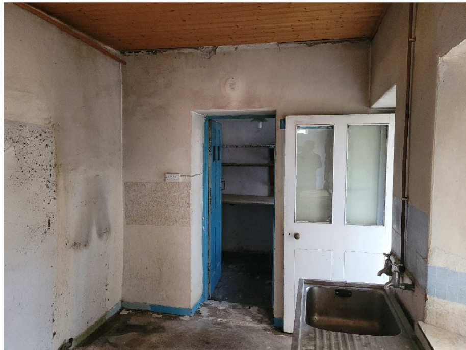
Wall between kitchen and pantry to be removed
