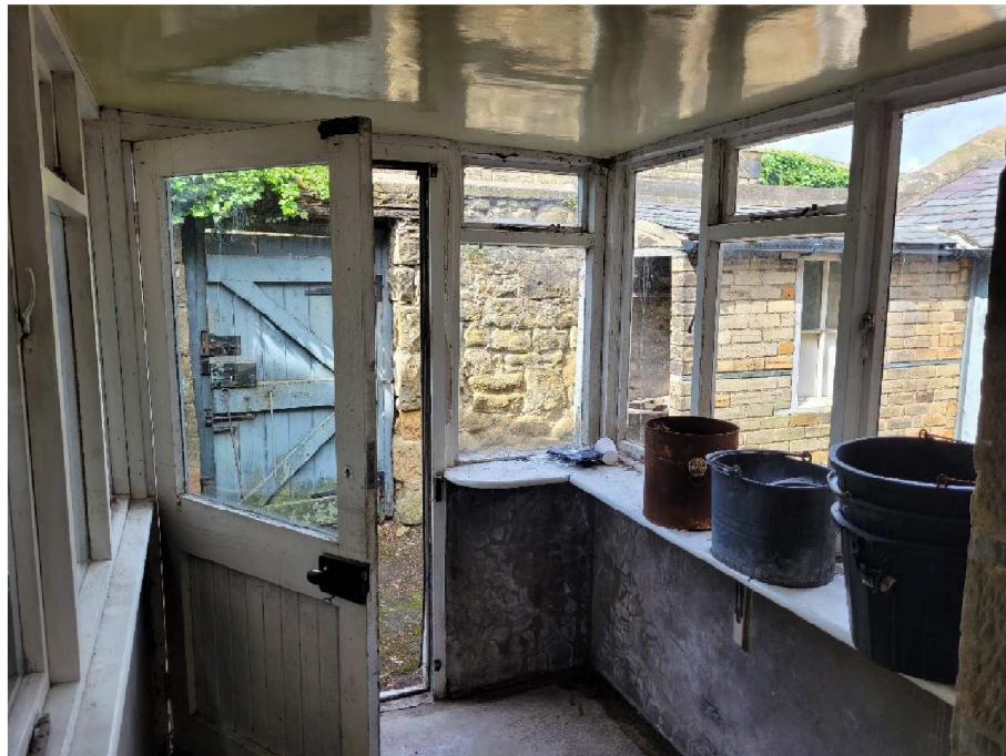
Non original timber porch to be demolished
