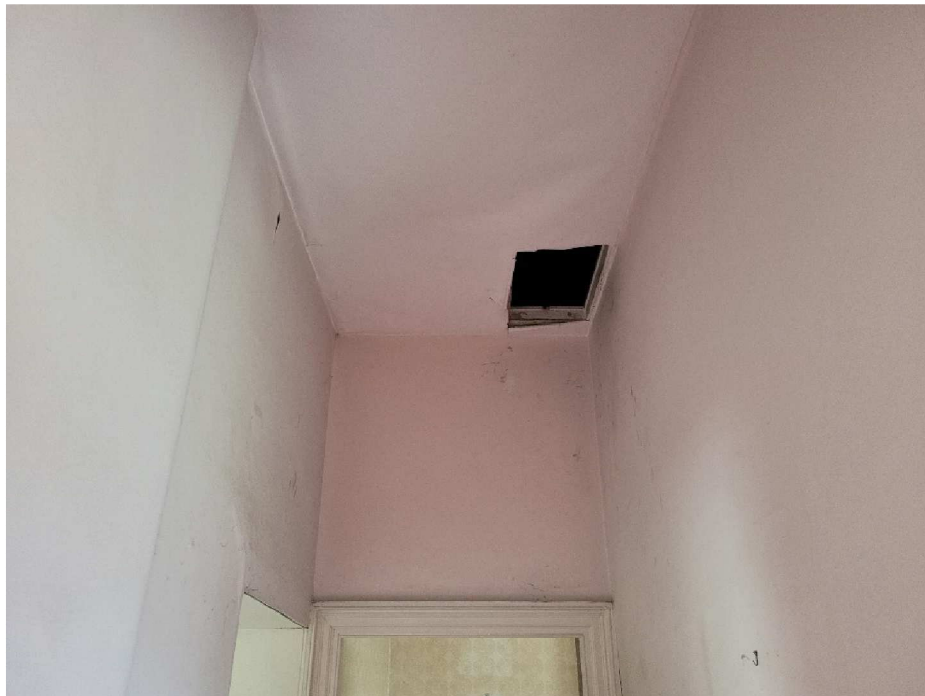
First floor landing. Enlarge existing trap hatch.
