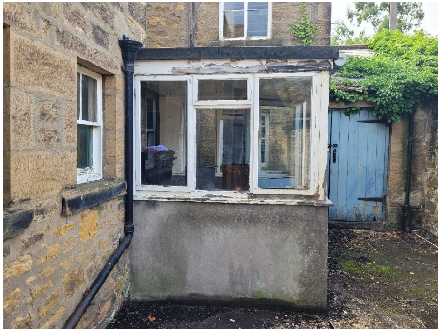
Non original timber porch to be demolished
