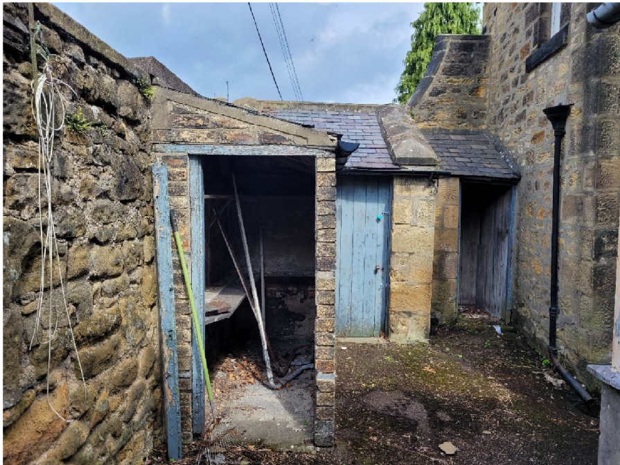
Non original outbuilding to be demolished
