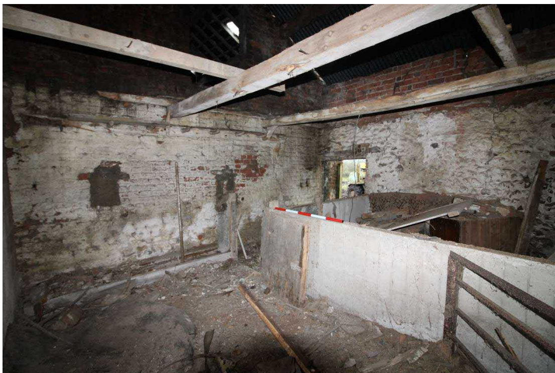
Plate 51: Southern extension, facing north-east with 1m scale
