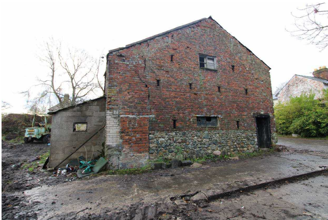
Plate 14: Northern gable elevation, facing south-west
