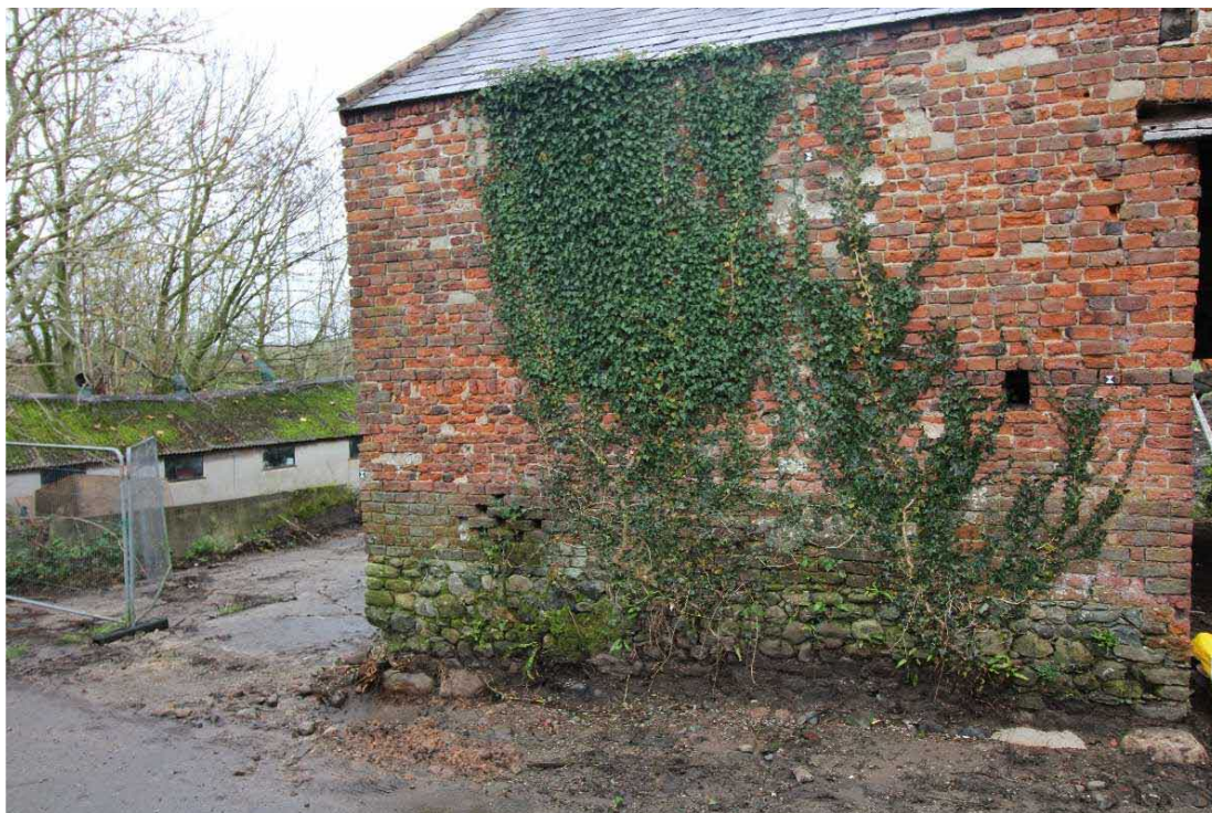
Plate 12: Cobble construction of lower wall, with secondary phase above partially obscured by vegetation, facing north-east
