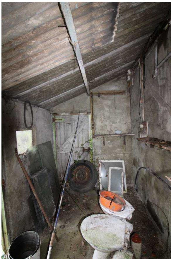
Plate 23: Interior of Lean-to structure, facing south
