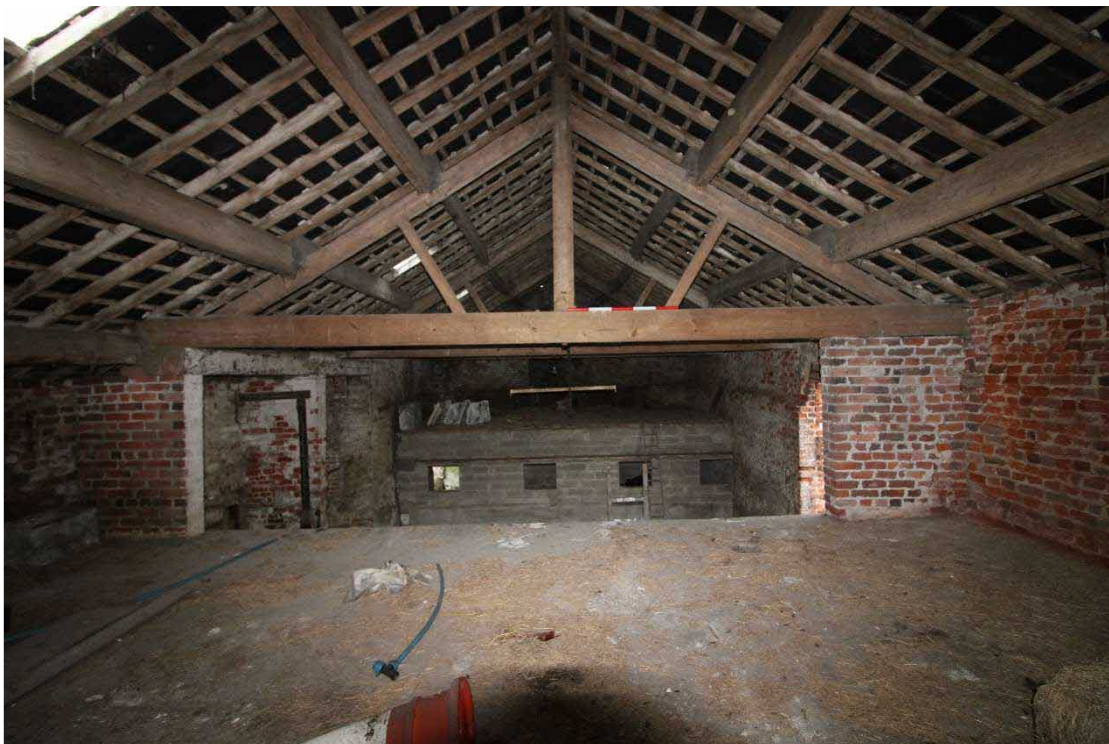
Plate 48: Northernmost King post truss, facing south, with 1m scale
