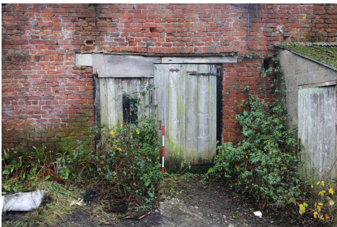
Plate 21: Eastern cart entrance, with soldier course to left at lintel height. Facing west with 1m scale
