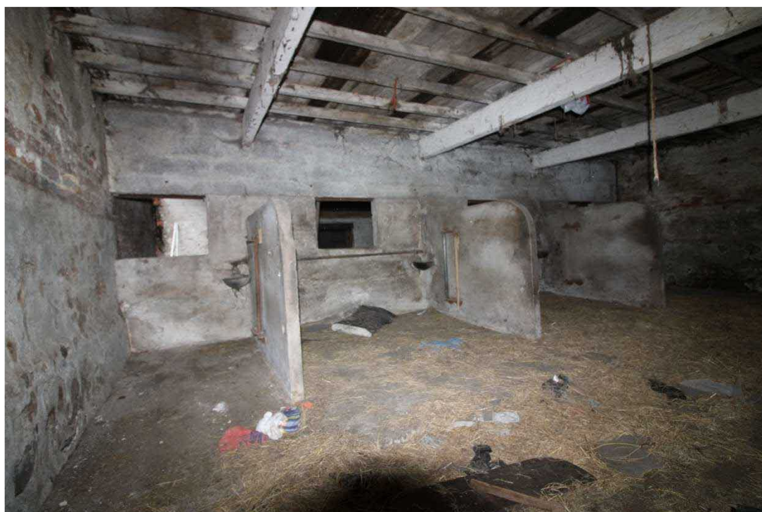
Plate 39: Southern byre, showing single stall to left of frame and double stalls to centre and right
