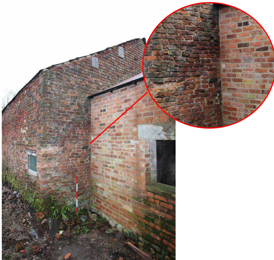
Plate 27: Southern gable elevation, showing fossilized pitch of original roof line. Facing north-east with 1m scale
