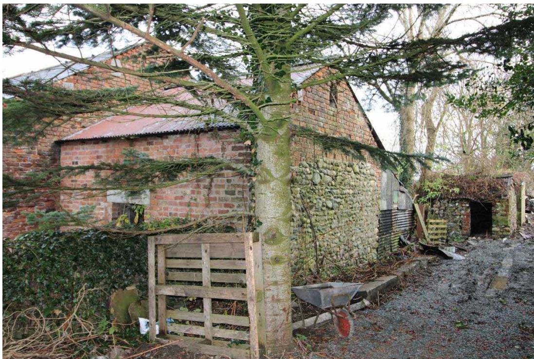
Plate 31: Southern extension, showing southern gable to right of frame. Facing north-east
