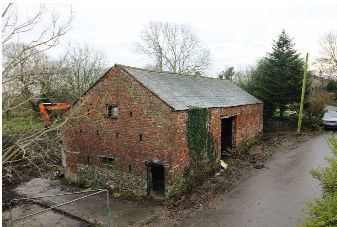
Plate 7: Barn from the north, facing south-east
