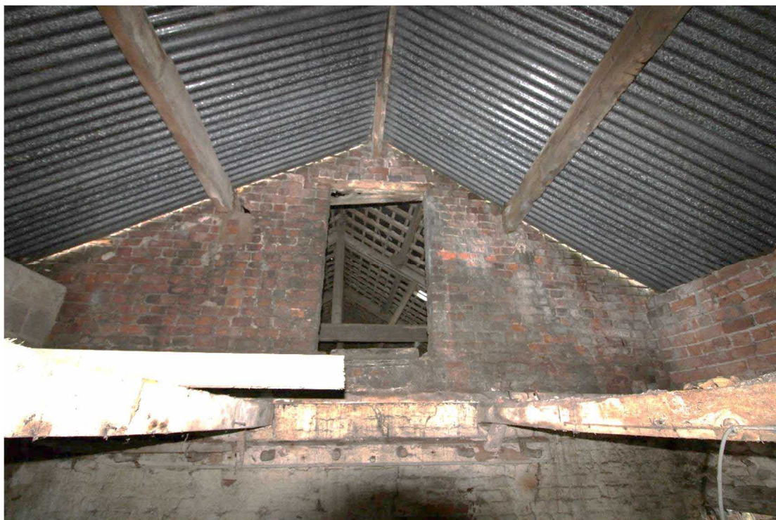
Plate 29: Loading door at centre of southern gable. Facing north
