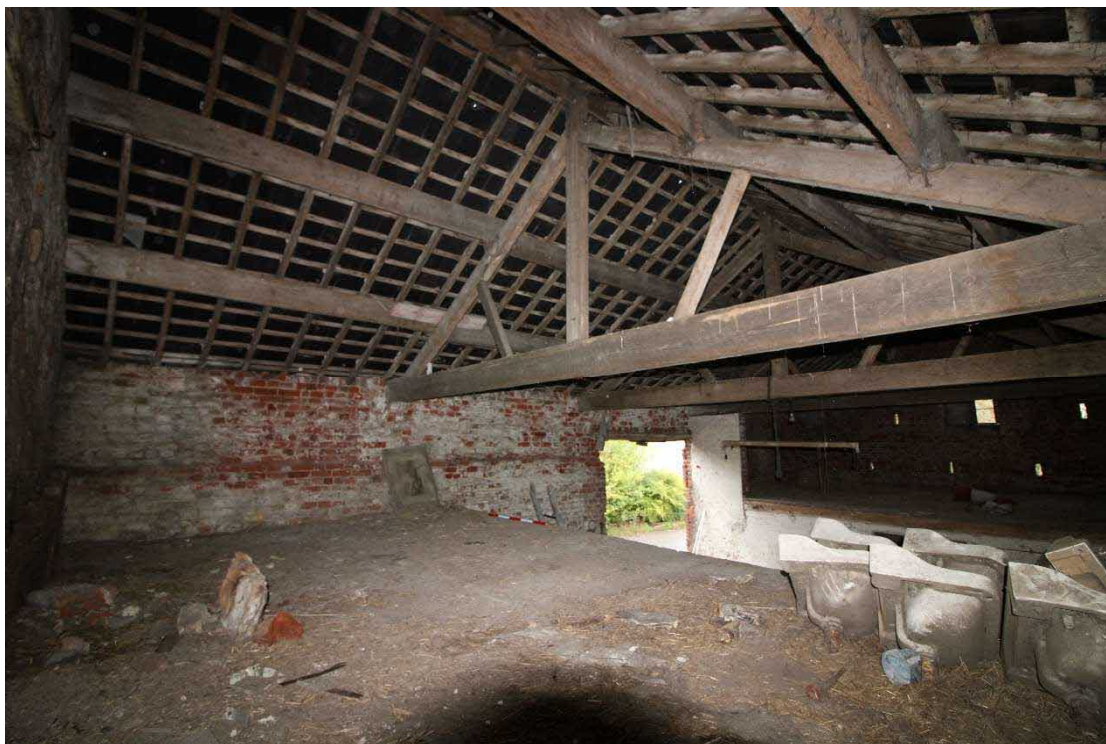
Plate 46: Southern mezzanine, facing north-west
