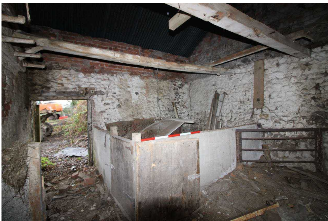
Plate 52: Southern extension, facing south-east with 1m scale
