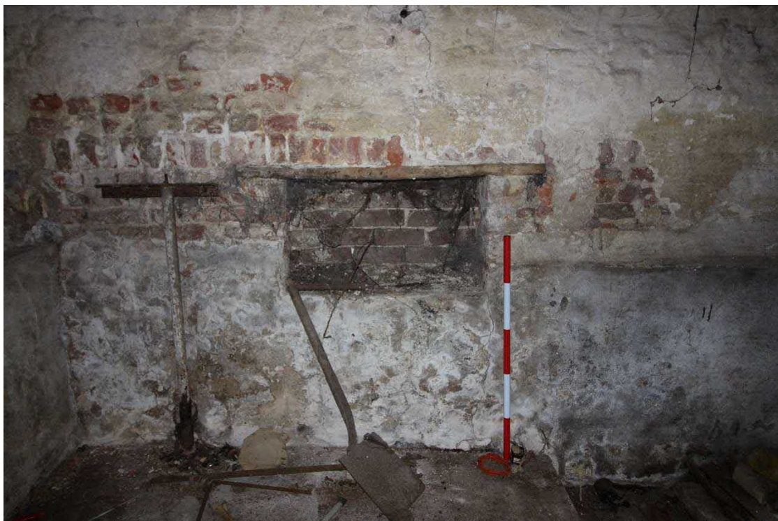
Plate 36: Recess at centre of western wall, Facing west, with 1m scale
