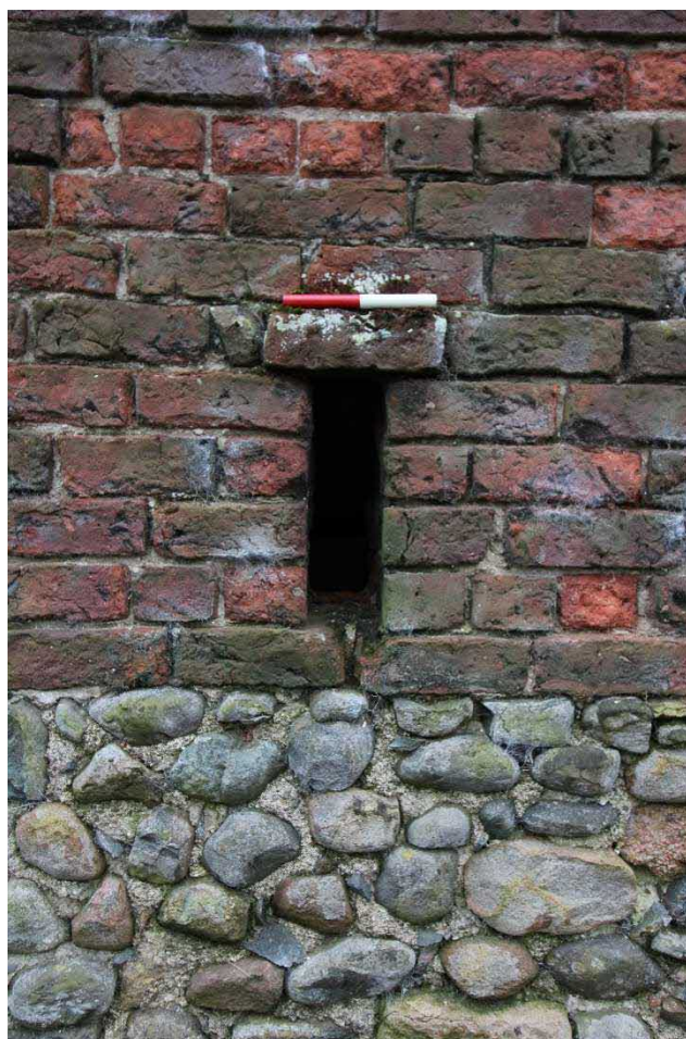
Plate 19: Ventilation loop on northern elevation. Facing south with 0.2m scale
