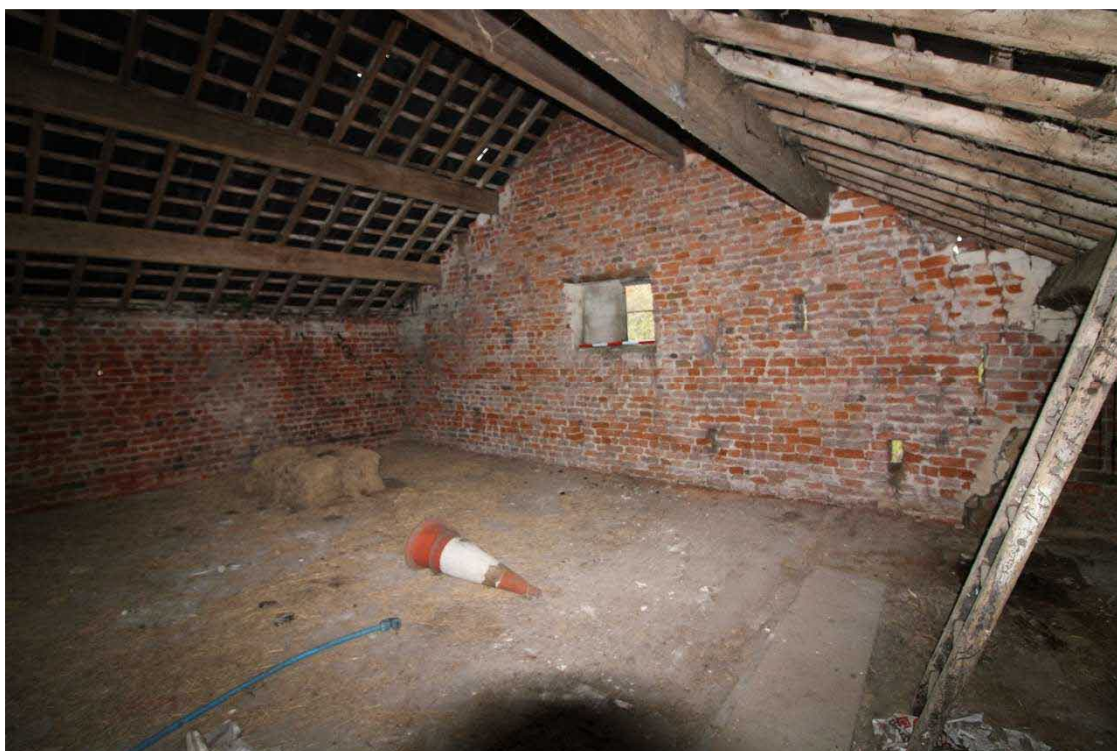
Plate 45: Northern mezzanine, facing north
