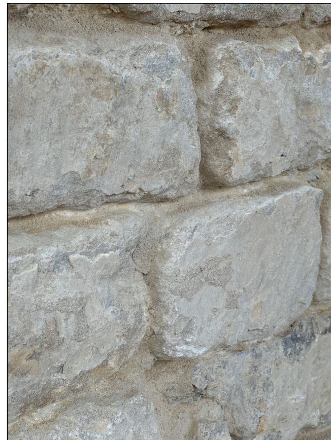
EXPOSED STONEMWORK (SAMPLE UN POINTED)
