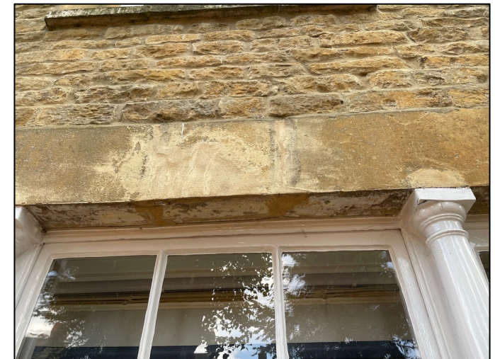
Figure 3: Examples of the stone replacements to the front window surrounds.
