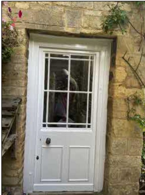
A western doorway provides access into the rear range from the garden. The flanking walls exhibit different characters; coursed rubble to the north and squared and dressed to the south. The timber-door itself comprises four-glass panes with margin lights (coeval to the ground floor window) and two –panels below set in timber architrave, underneath a dressed stone lintel with keystone wedge (Fig. 9).
