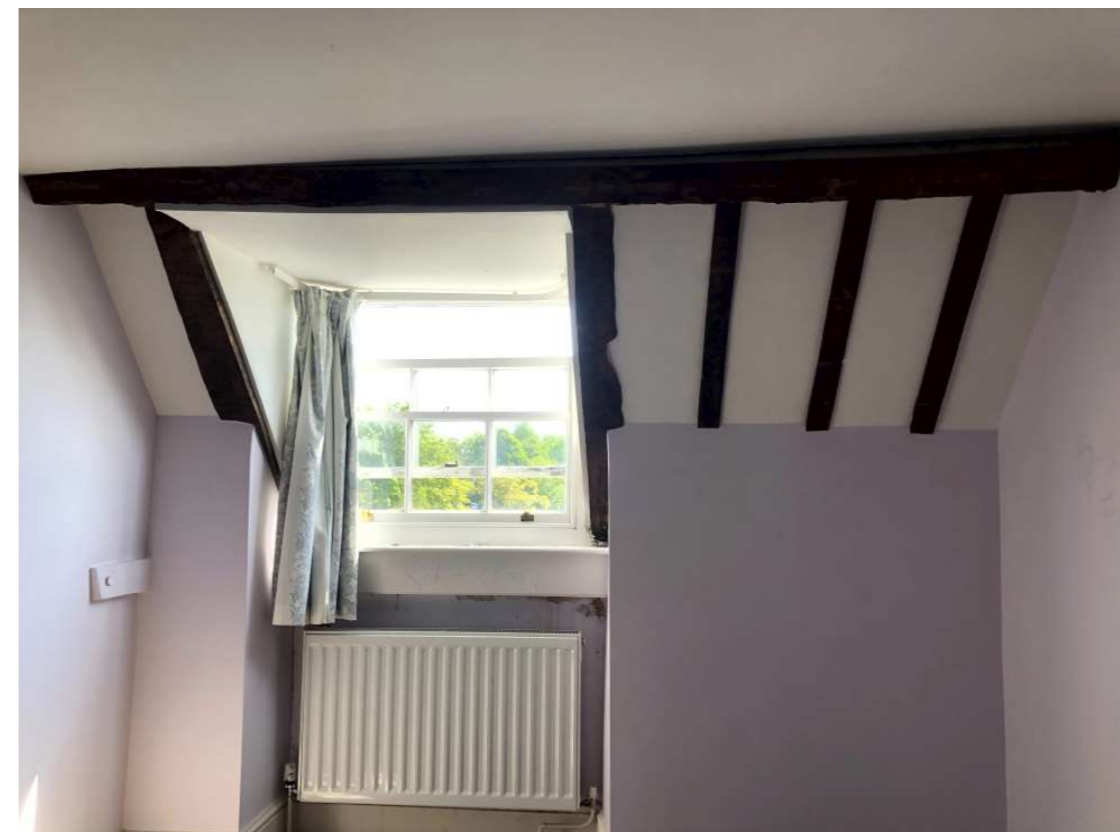
Second Floor rafters
