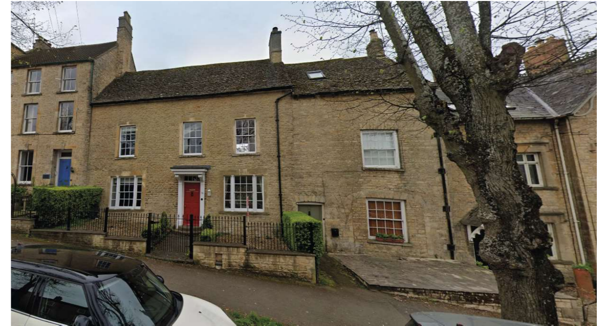
Street Facing Facade (North)
