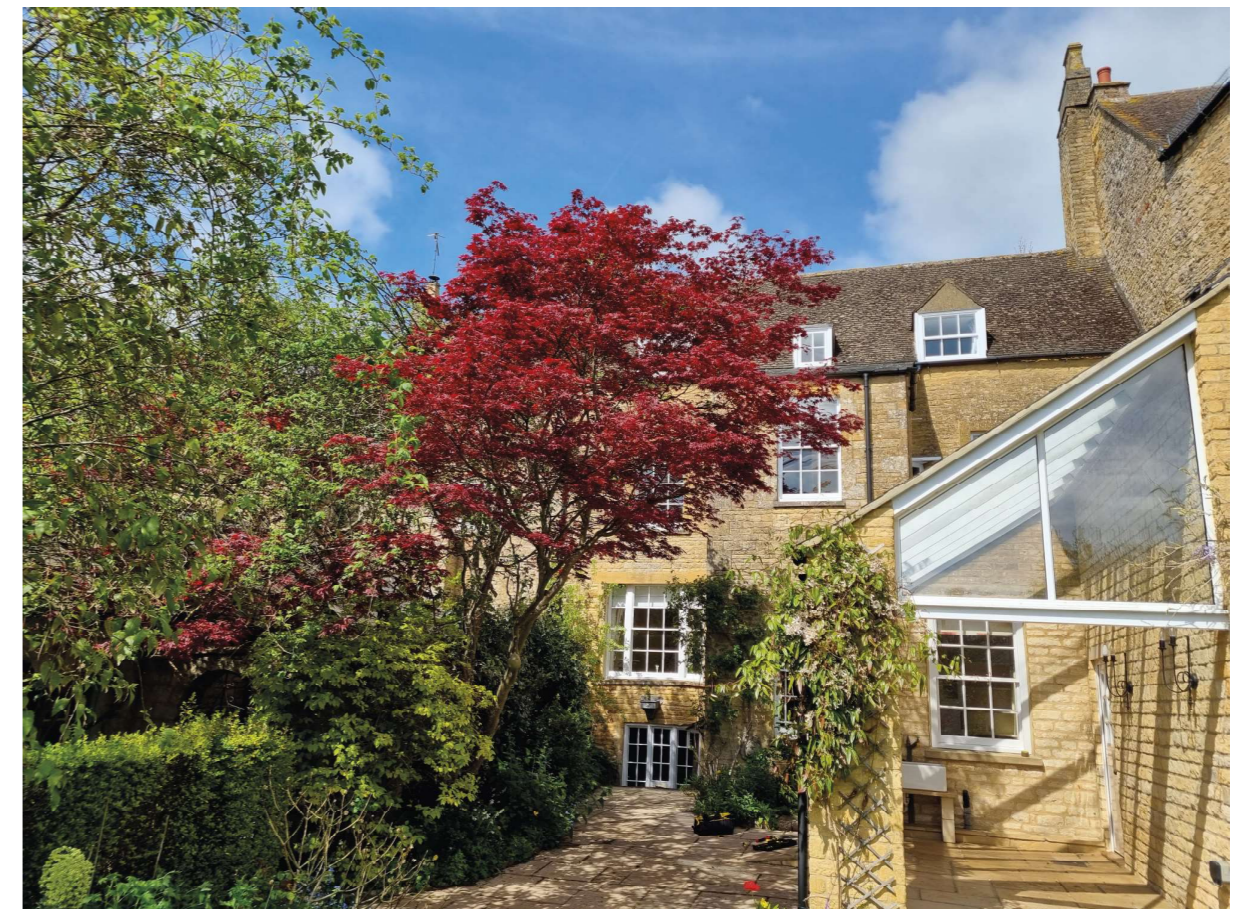
Rear Facade (South) - Window to lower ground floor bottom left
