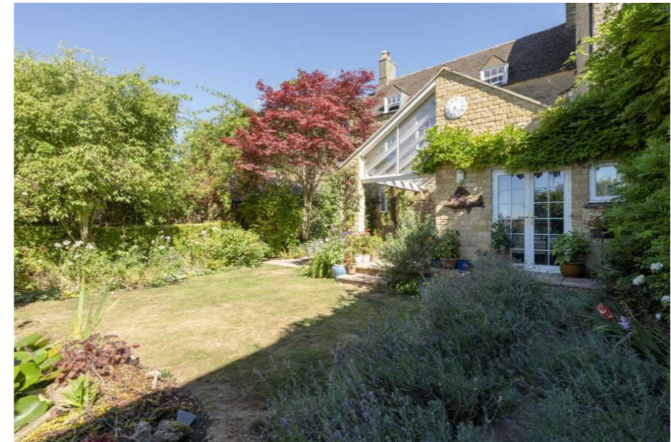
View of existing extension from the garden
