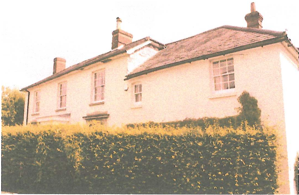
Figure 5 Front elevation from the street.
