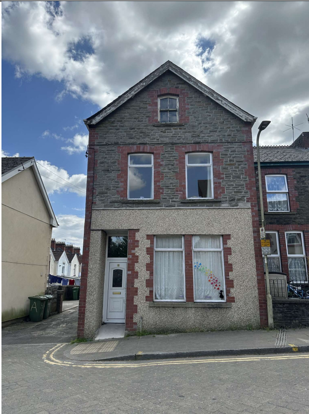
Front view-principal view - North
