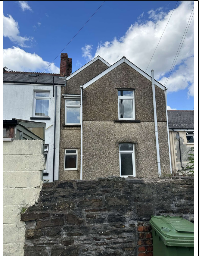
Rear view - South
