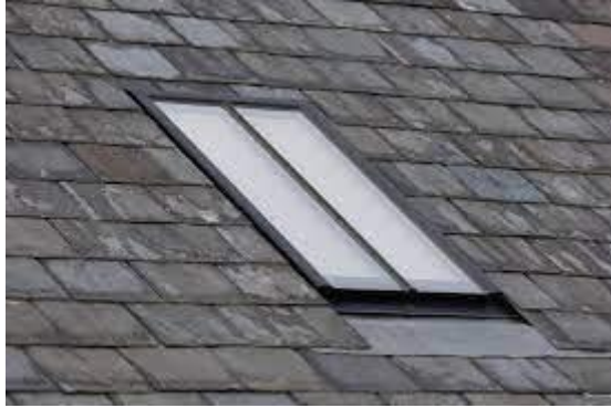
Conservation rooflights fitted flush
