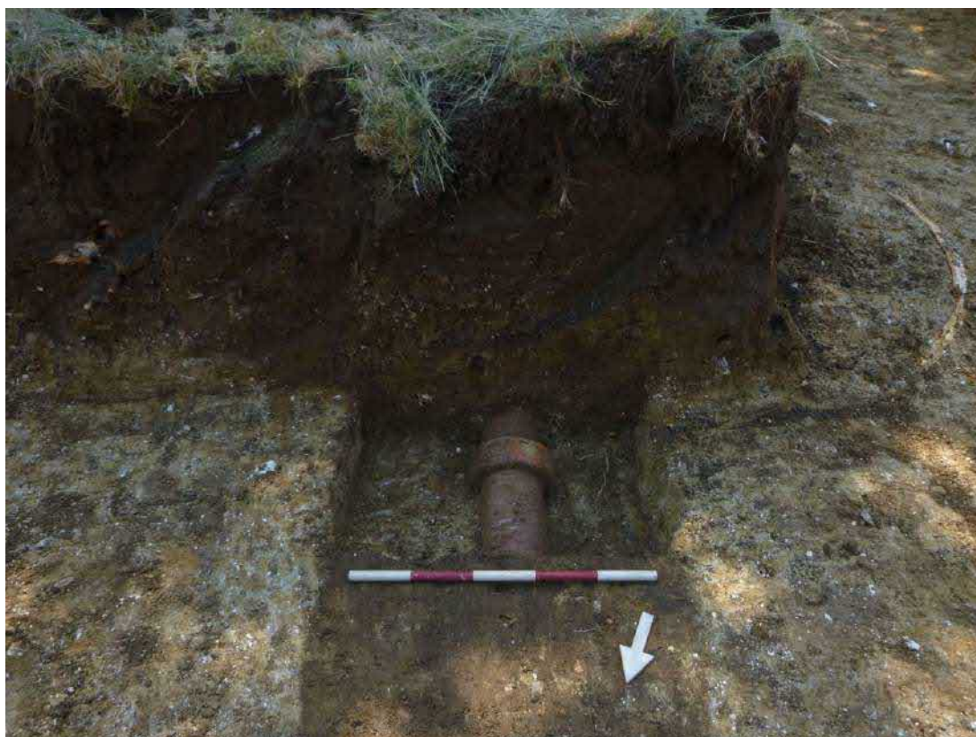
Photograph 4 Modern service in T1, looking south south-east.
