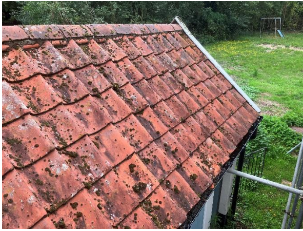
Photo 15: Closely fitting tiles of rear shed
