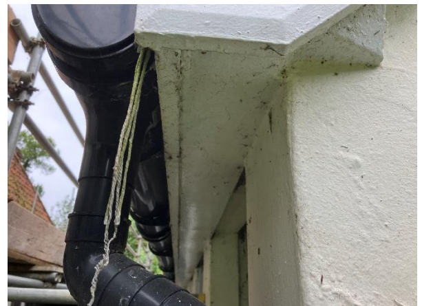
Photo 14: Closely fitting soffits and barge board of rear shed
