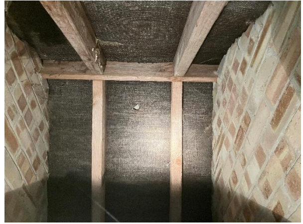
Photo 16: Internal view of rear shed
