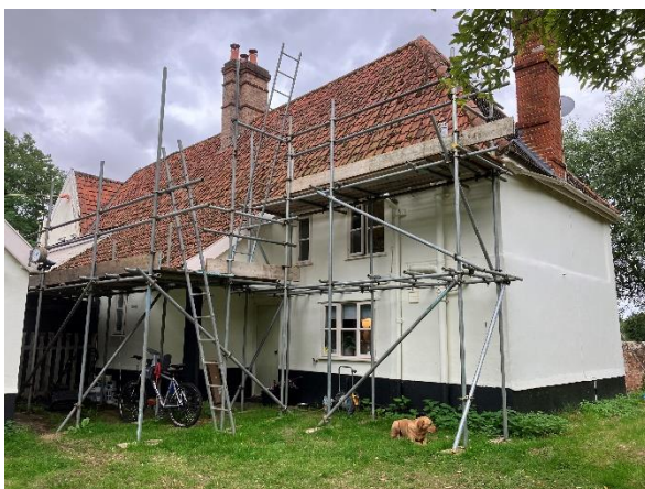
Photo 1: North western facades of farmhouse
