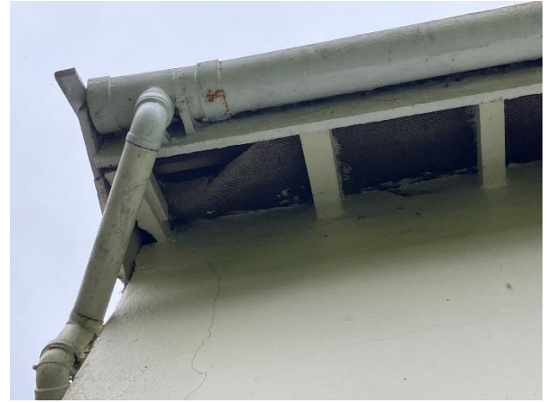
Photo 4: Potential bat and bird access point around eaves of farmhouse
