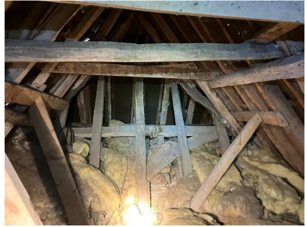
Photo 10: Eastern end of loft space, where floor is raised
