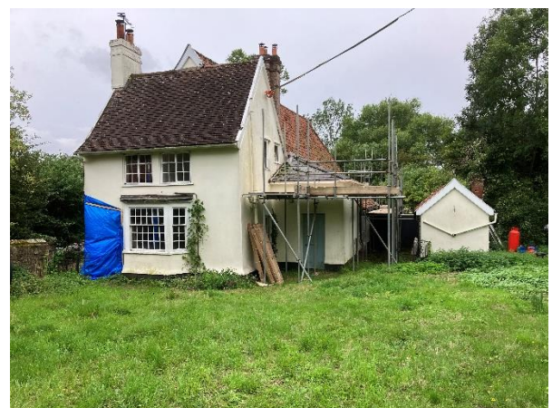
Photo 2: Eastern facades of farmhouse and rear shed
