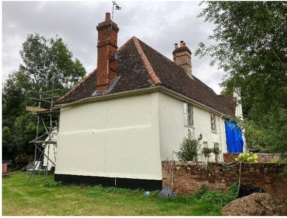
Photo 3: South western facades of farmhouse
