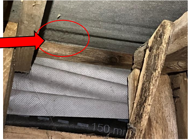
Photo 22: Likely location of roosting bats indicated by piling and pulling of roof membrane fibres
