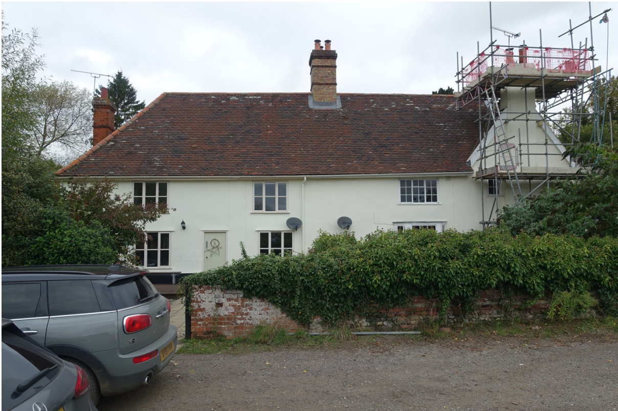
Picture 3 – The front elevation of (No's 1 & 2) Lime Kiln Farmhouse.
