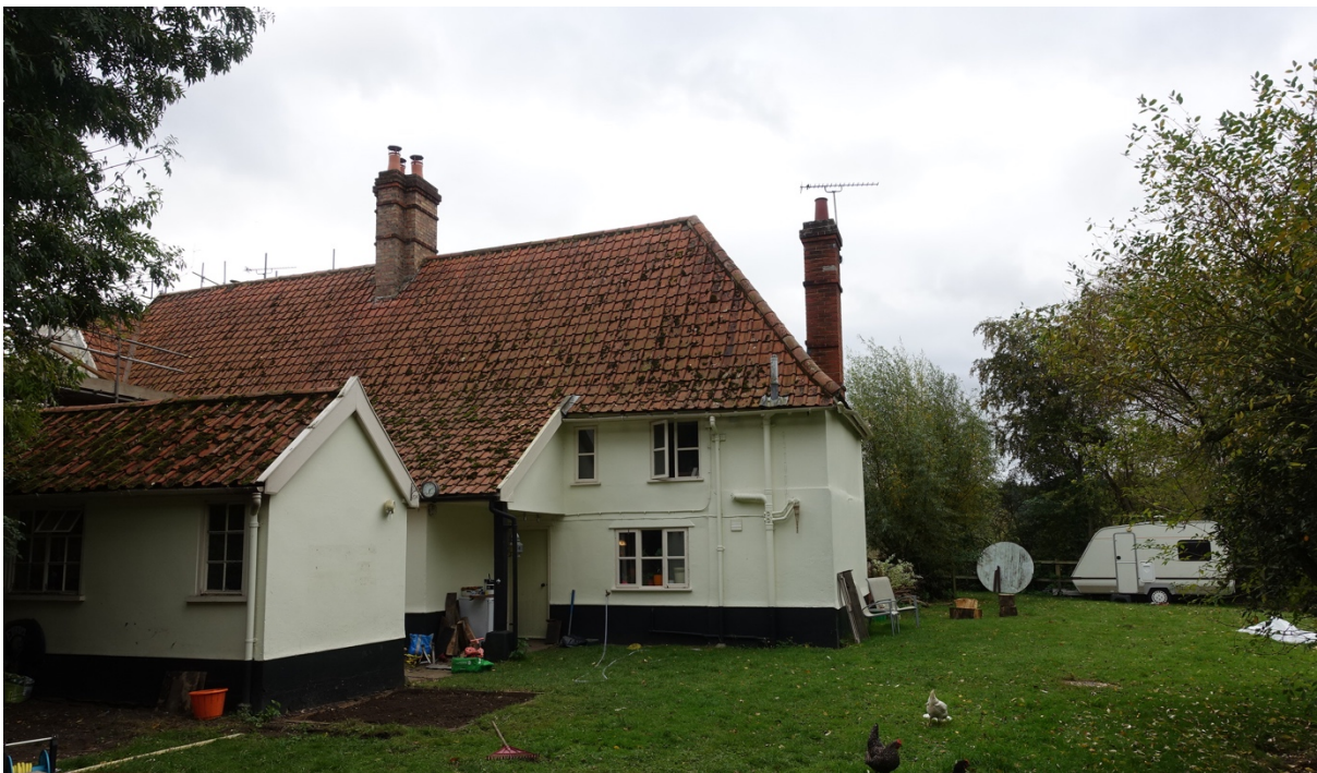
Picture 4 – The Rear elevation of (No.2) Lime Kiln Farmhouse, & detached outbuilding.
