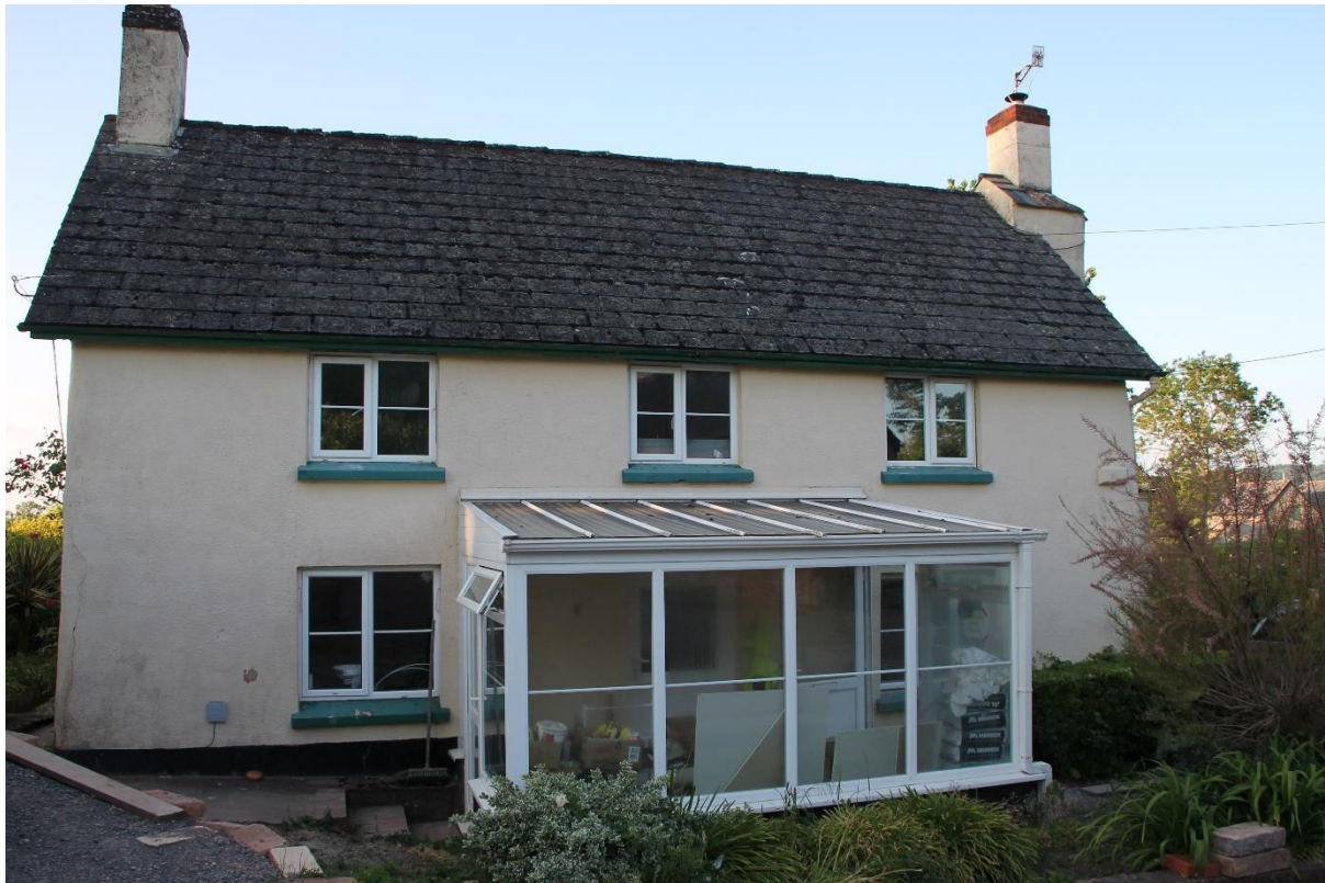
Photograph 1: showing a view of the target building
