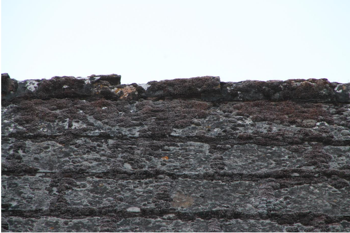
Photograph 3: showing the external roof structure
