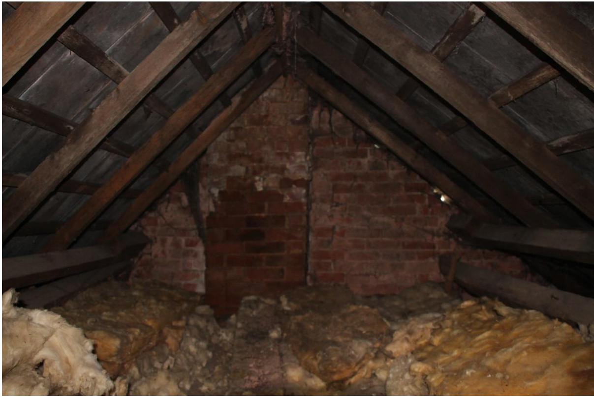
Photograph 5: showing an internal view of the loft space
