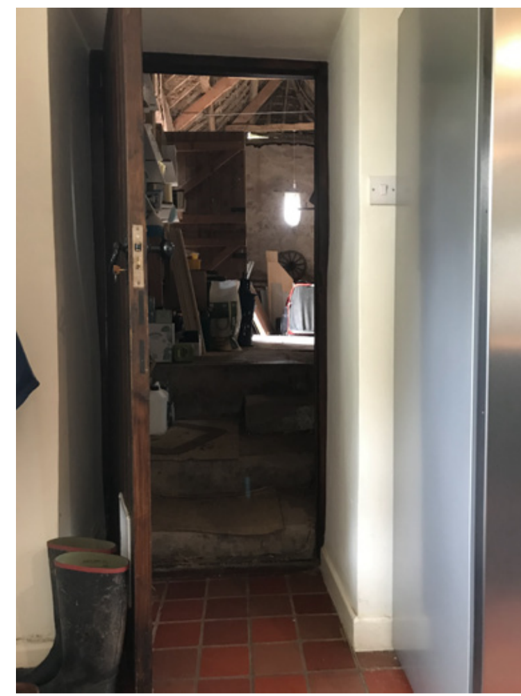
Existing steep concrete steps from Cottage to Threshing Barn
