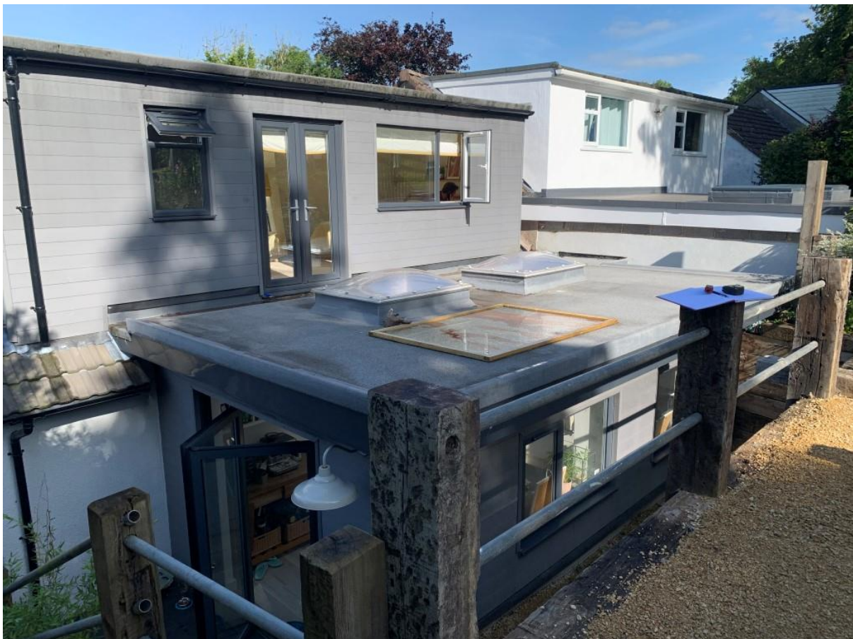
Photo 2. The Rear of the House.
