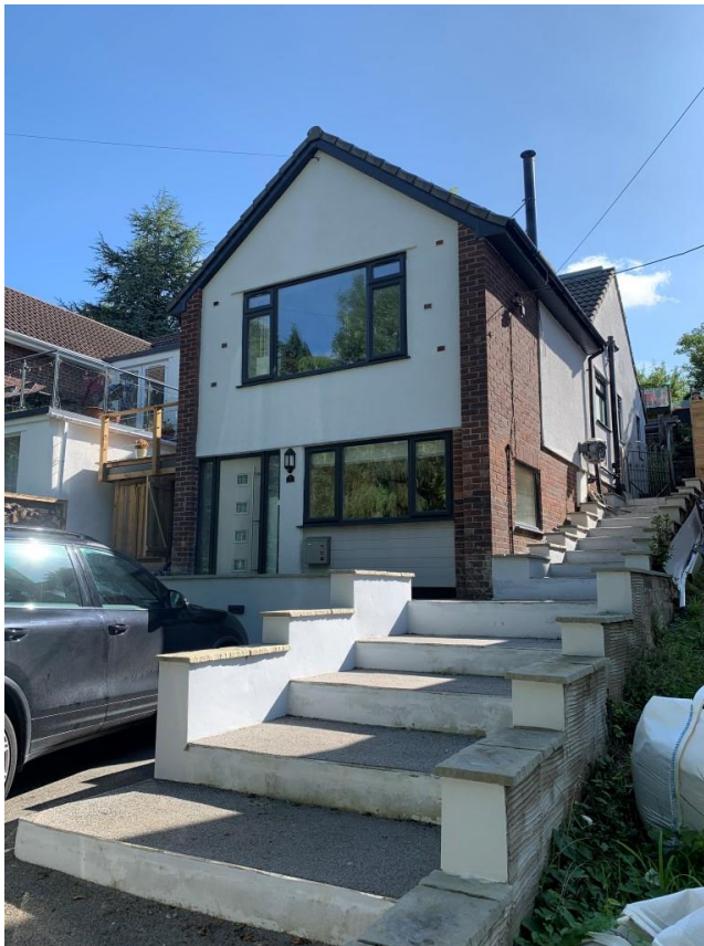
Photo 1. Existing Front Elevation. No works carried out to Front
